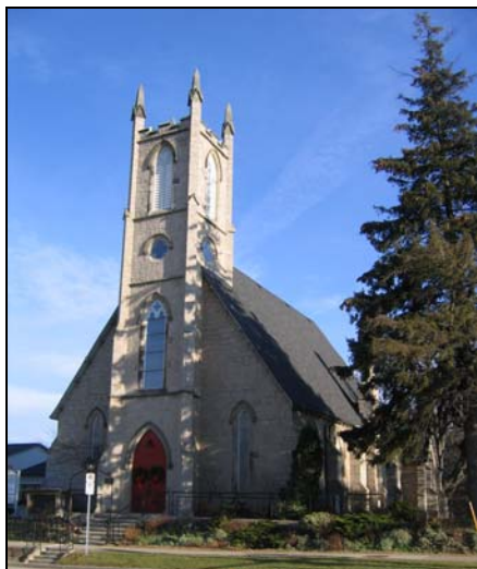
Fig.7 St. John's Anglican Church (1869), Ancaster
