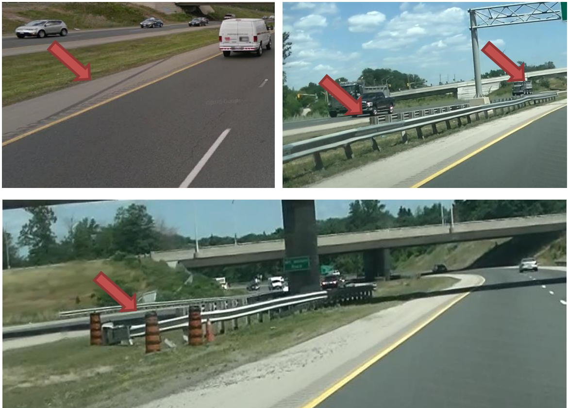
Figure 17: Evidence of loss of control towards the median / collisions with guide rails
