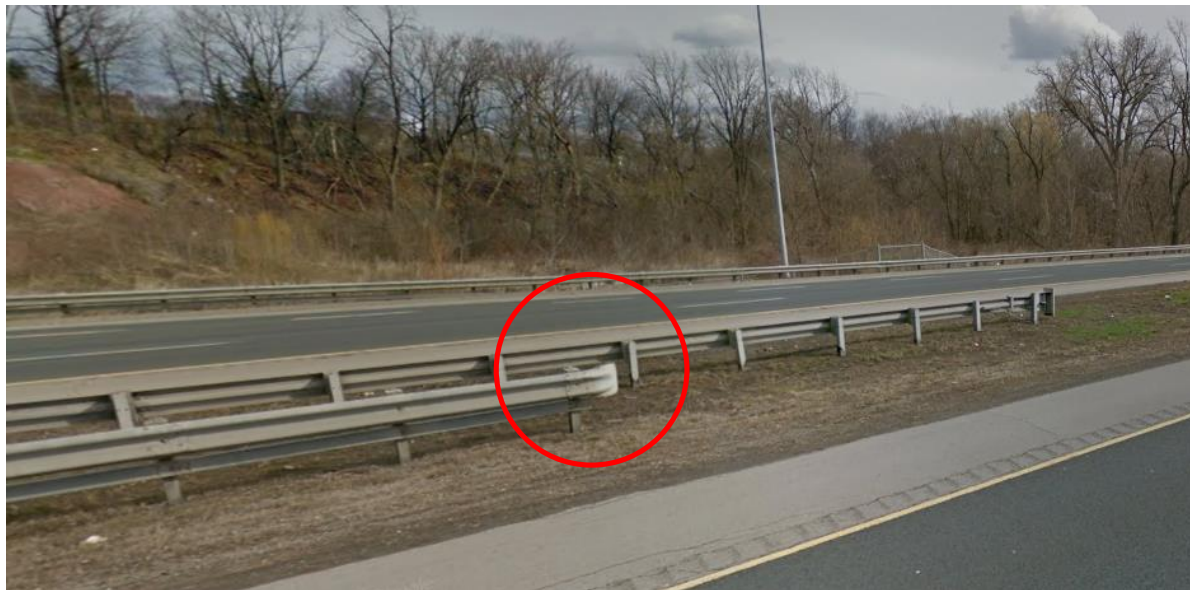
Figure 18: RHVP typical guide rail leaving end treatment
