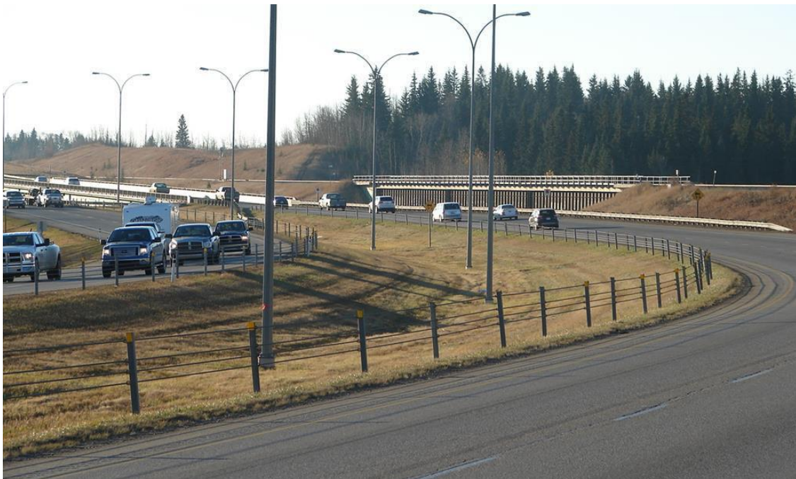
Figure 31: Example of high tension cable barrier
