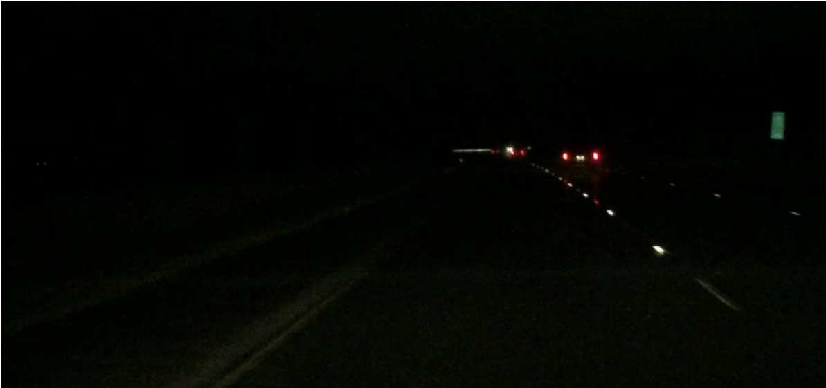
Figure 27: Pavement markings during nighttime condition (with PRPMs)
