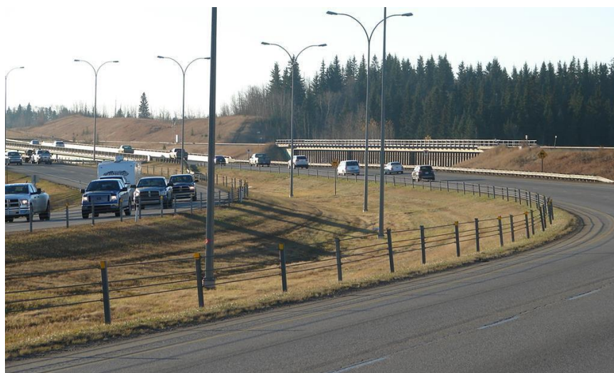
Figure 2 : An Example High Tension Cable Barrier
