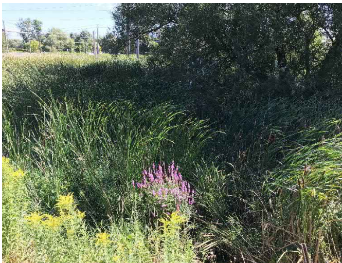
Photograph 27. ↑ WC-06. Downstream of culvert outlet facing downstream (east)
