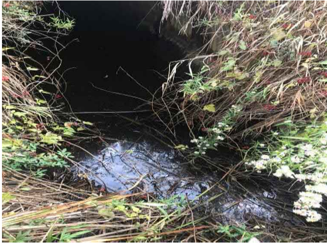
Photograph 25. ↑ WC-09. Water present at culvert inlet
