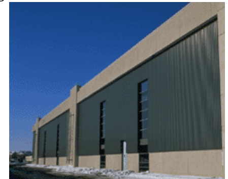
Solar Wall, Ford Plant in Oakville, ON
