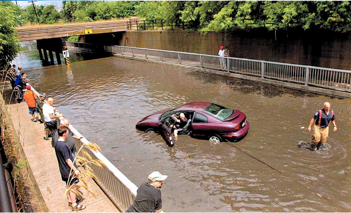
Kenilworth Ave. underpass
