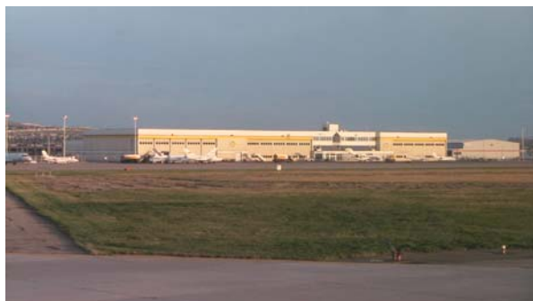
Calgary's Shell Aerocentre is the largest FBO/GA Facility of its type in Canada and is used as a home base for Regional Jet services by energy company aircraft . . . (Source: LPS AVIA)
