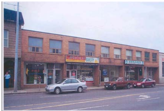
669 Barton Street East – Before
