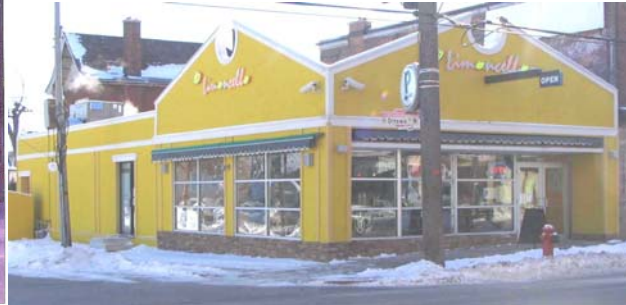
226 Ottawa Street North – After
