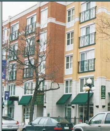
Mixed Use Building, Ottawa, Ontario
