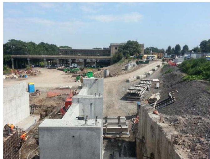
James Street North GO Station Under Construction
