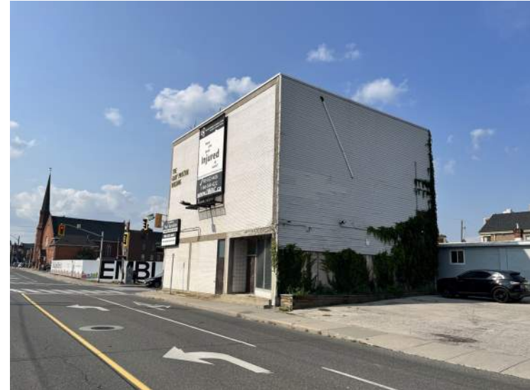
View of 92 John Street North (Gary Procter building) and adjacent parking lot, at the southwest corner of John Street North and Wilson Street. The adjacent development site at 41 Wilson Street is visible to the west, as is 37 Wilson Street - St. John's Evangelical Lutheran Church.
