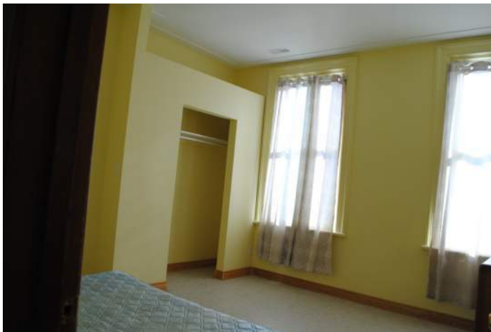
View of 81 Wilson Street, 2nd level interior. Both interior levels have been extensively altered for residential use. Pictured above is a bedroom on the second level.
