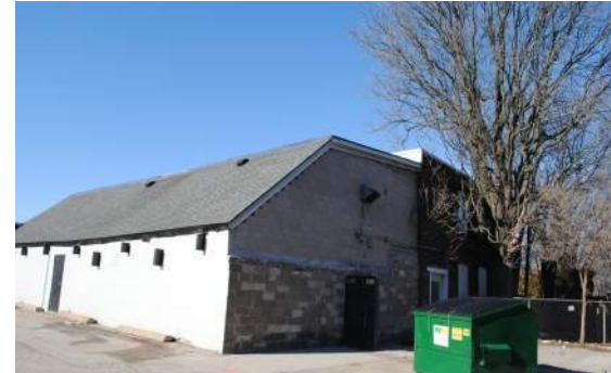
Eastern addition of 98/100 John Street North, looking west. The presence of imperial sized cinder blocks suggests that alterations were undertaken on the rear wall before the 1960s.
