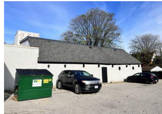
Eastern addition of 98/100 John Street North, looking north.
