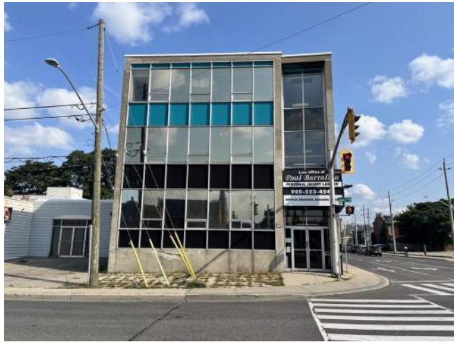
View of development site looking east from the west side of John Street North at the intersection of Wilson Street. The curtain wall of 92 John is visible here, and a portion of 96 John Street to the north.
