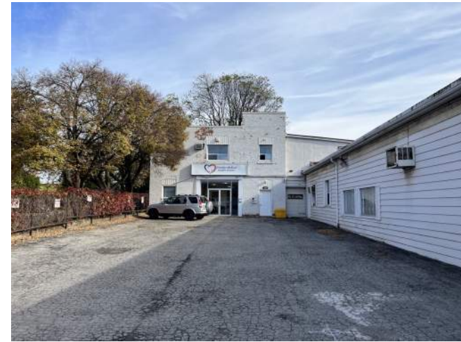
View of 100 John Street, looking east from John Street. The original building is set back from the street by approximately 30 metres with a linear addition clad in vinyl visible to the south, both of which were most recently occupied by a framing studio.
