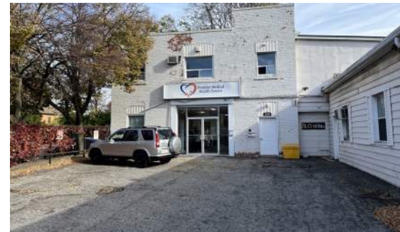
100 John Street North, looking east.
