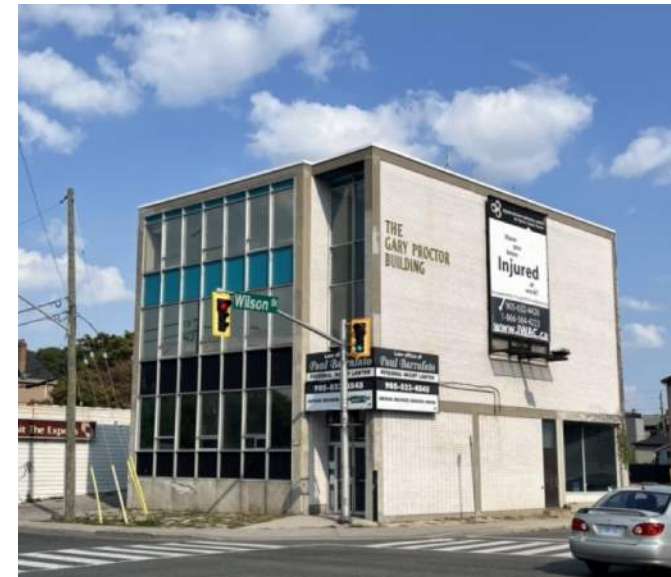
View of 92 John Street North, looking northeast from the south side of Wilson Street.
