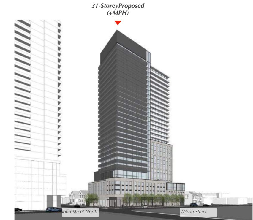
East Elevation - Looking north-east towards the subject development site. Numerous set-back and setbacks have been added to the massing of the tower, supplanting the 5 storey podium on Wilson and John St. N (16.0m high on both sides, below the permitted 22m height). This includes the introduction of a mid-rise form on east side to transition from low-rise/podium level to tower. On the east wall a 5-storey podium faces adjacent building (16.0m high), with a change in materials and articulation to improve the relationship with the existing context. The modest height increase between the adjacent heritage buildings to the north (144 John Street) and to the east (87 Wilson Street) is sympathetic to the heritage resources, and will exemplify human scale development in light of the addition of a large tower above into the historic context.
