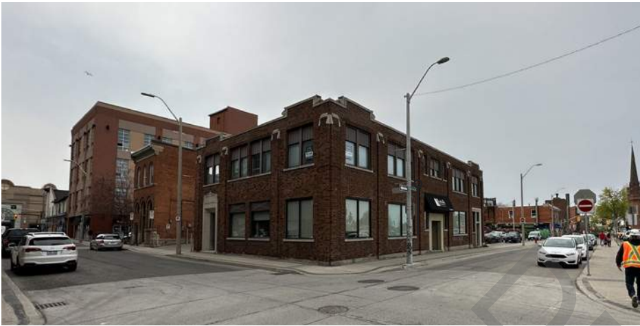
Figure 24. View of the Heritage Property located at 69 Rebecca Street from Hughson St. N and Rebecca St. intersection looking northwest
