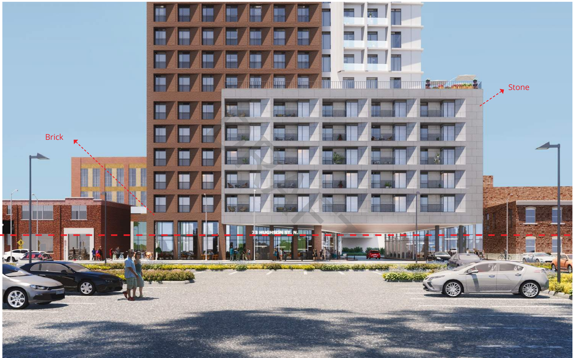
Figure 49. Rendering of the proposed Development showing the proposed podium level incorporating the contextual materials and horizontal datum lines and the adjacent heritage resources at 69 Hughson Street and 30 Willson Street, mcCallumSather Architects June 2023
