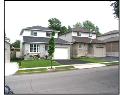
Infill: West 2 nd St., detached houses
