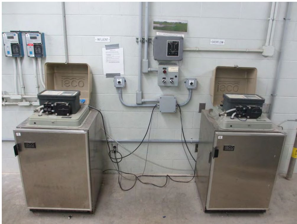
HCS04 – Sewage Lift Pump Nameplate
