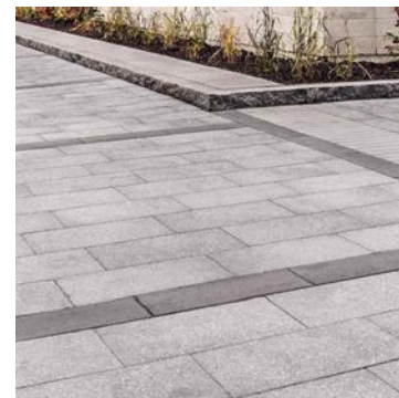
Precast Concrete Unit Paving
