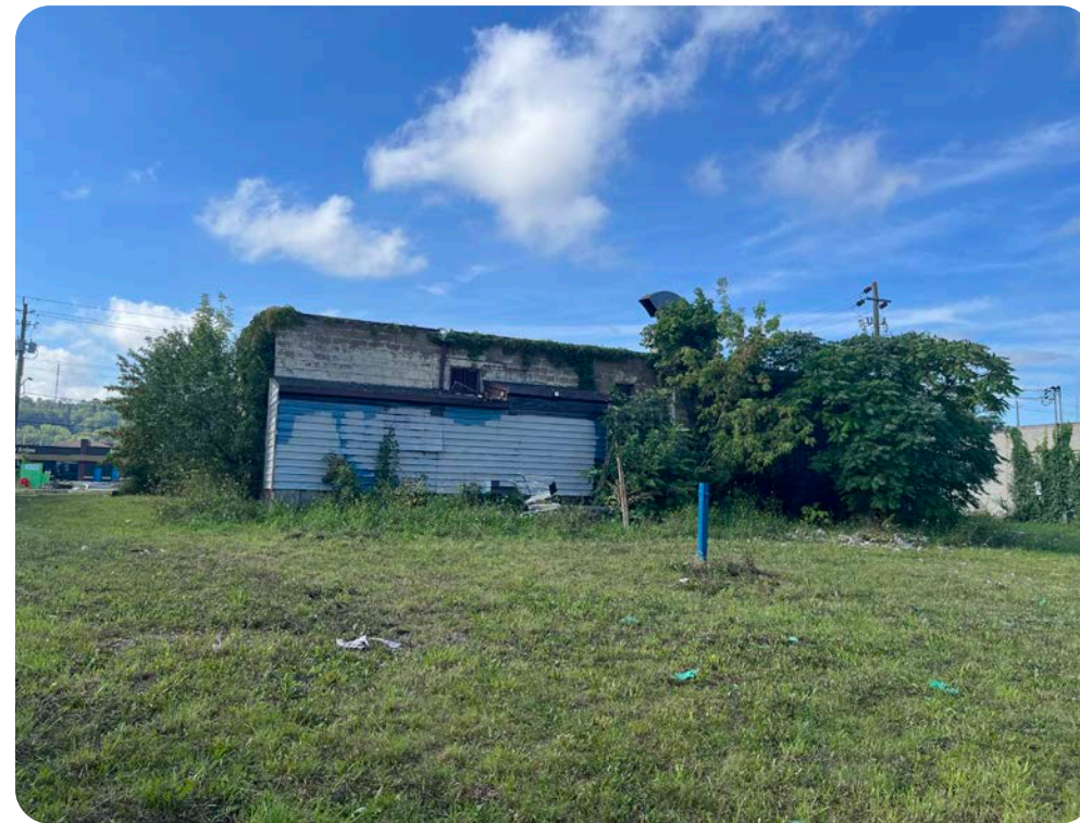
2. On the subject site looking south toward the rear of the existing building on site.
