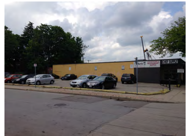
Under-utilized surface parking lots are key candidates as Opportunity Sites and redevelopment can significantly impact the public realm (Top: parking lot at north west corner of James St N and Colbourne St. Bottom: parking lot at north west corner of James St N and Murray St.)
