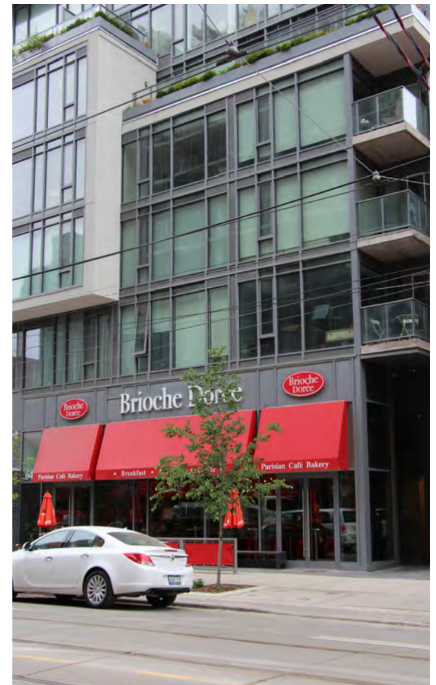
Building articulation provides interest in the streetscape
