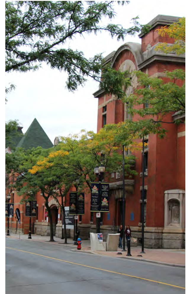
John Weir Foote Armoury, an important cultural heritage site in the Study Area
