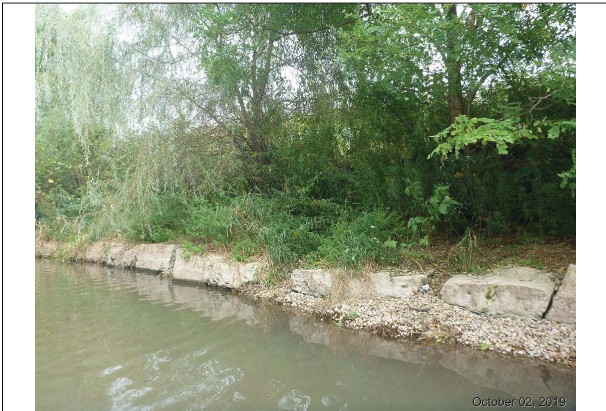
Photograph 2. Riparian bank edged with armour stone along Chedoke Creek.
