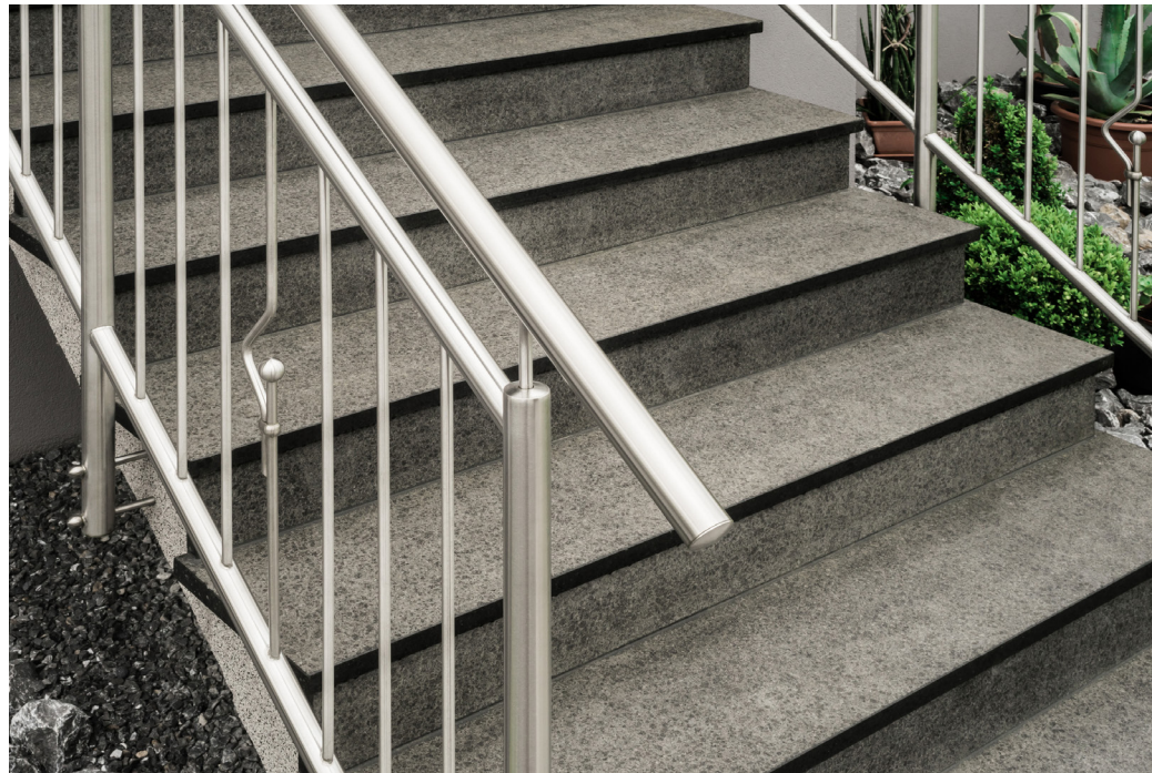
04 EXISTING STEEL STAIRCASE CLAD WITH NON-SLIP GRANITE TREAD
