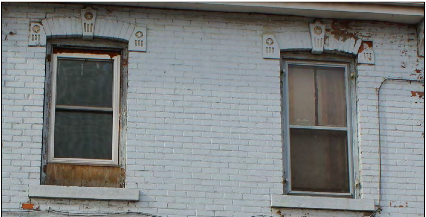
Photograph 8: View showing details brick segmental arch lintels and concrete details on rear portion of 563 King Street East building, formerly 3 Steven Street (AECOM, 2017)
