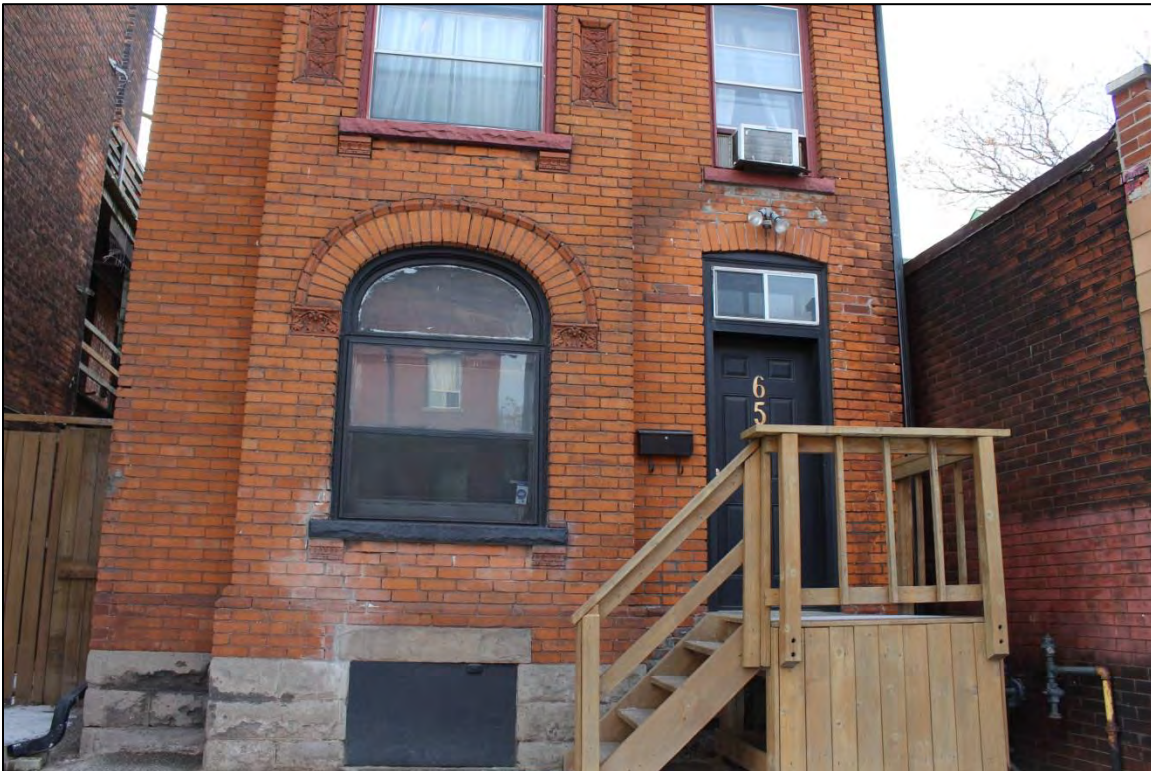
Photograph 2: Details of window sills and basket arches articulated by an edging around the voussours on the main floor of 656 King Street East (AECOM, 2017)
