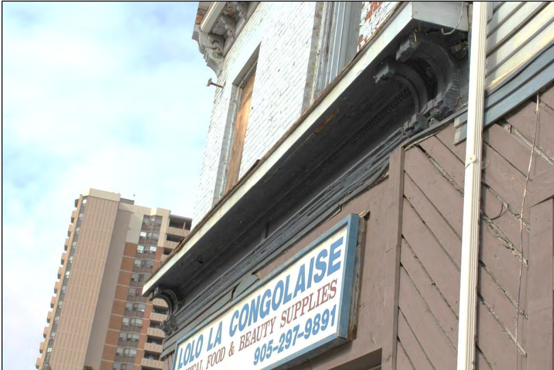
Photograph 5: View showing cornice and bracket details between ground floor and second storey (AECOM, 2017)
