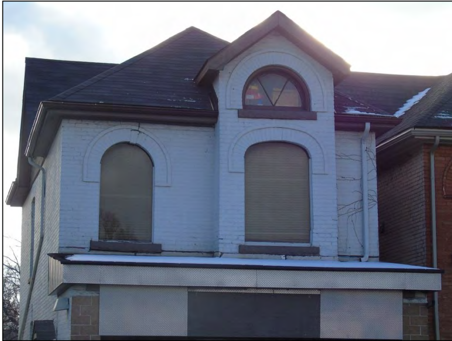
Photograph 5: Second storey details including arched brick lintels, concrete sills, and round-headed attic window
