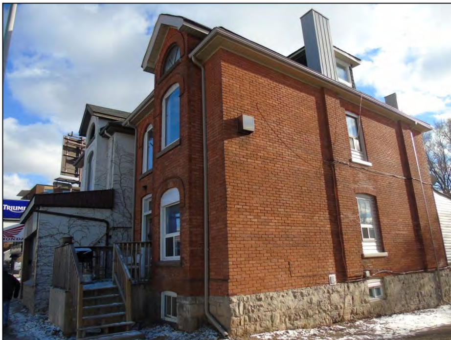
Photograph 4: View showing west facade of 621 King Street West, showing rubble stone foundation and smooth exterior brick
