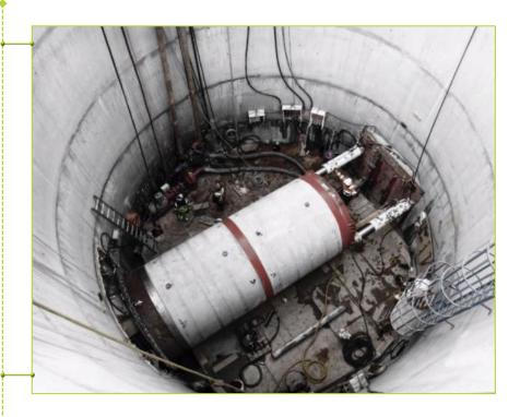
In other sections (for approximately 7.5km), the deeper vertical alignment of the sewer and/or ground conditions present make open cut construction challenging or impractical. Therefore, tunneling construction methodology will be employed to minimize social and environmental impacts.
