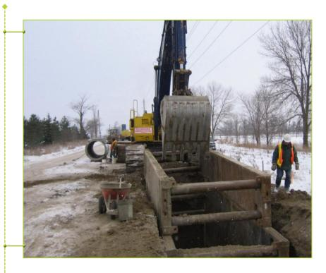
Due to relatively shallow depths (up to 8m), open cut construction method is planned to be used for a portion of the sanitary trunk sewer along Dickenson Rd. extending 2.5km± from Upper James Street to just west of Miles Rd as well as a local watermain.
