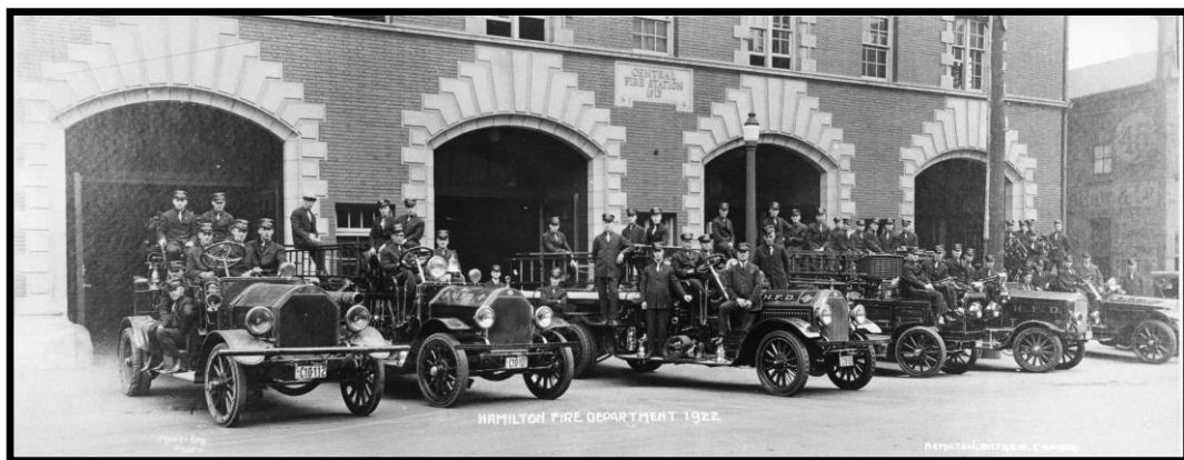
Central Fire Station -1922
