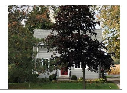
Foundation: Construction Material: (Wood-frame) Cladding: Siding (horizontal) Roof Type: Gable (Side) Roof Material: Asphalt
