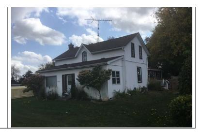
Foundation: Construction Material: (Wood-frame) Cladding: Siding Roof Type: Gable (Side) Roof Material: Asphalt
