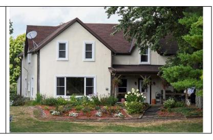
Foundation: Construction Material: Wood-frame Cladding: Stucco Roof Type: Gable (Cross) Roof Material: Asphalt
