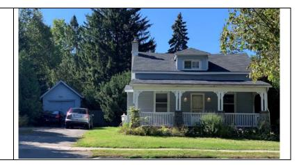
Foundation: Construction Material: (Wood-frame) Cladding: Siding Roof Type: Gable (Side) Roof Material: Asphalt
