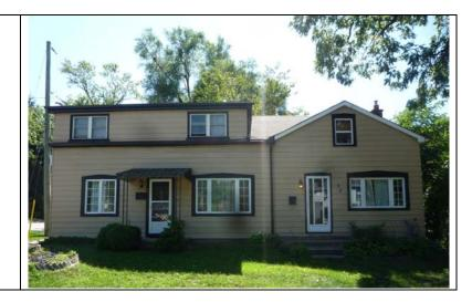
Foundation: Construction Material: (Wood-frame) Cladding: Siding Roof Type: Gable Roof Material: Asphalt
