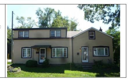
Foundation: Construction Material: (Wood-frame) Cladding: Siding (horizontal) Roof Type: Gable Roof Material: Asphalt
