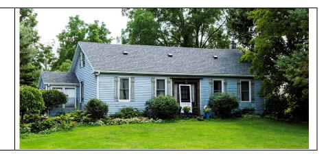
Foundation: Stone Construction Material: (Wood-frame) Cladding: Siding (horizontal) Roof Type: Gable (Side) Roof Material: Asphalt
