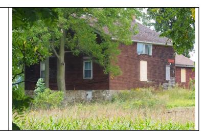
Foundation: Stone Construction Material: (Log) Cladding: Insulbrick Roof Type: Gable Roof Material: Asphalt
