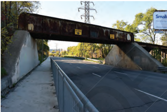
Plate 20: View of Birch Avenue Bridge looking southwest
