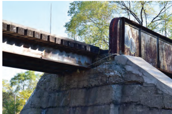
Plate 29: Close-up View of west abutment looking southeast
