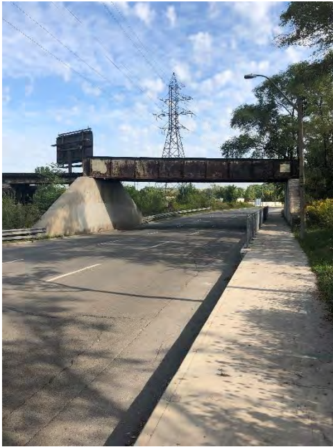
Plate 13: View of the centre bridge (Bridge 331) crossing Birch Avenue, looking north.
