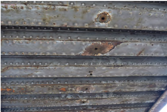
Plate 24: View of underside of bridge
