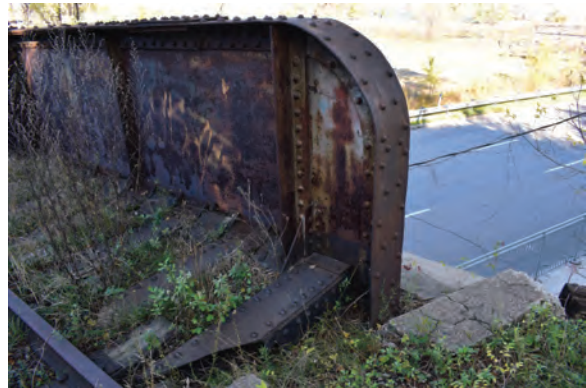
Plate 23: Close-up view of steel girder at northeast end
