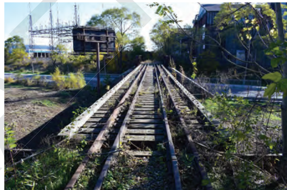
Plate 19: View of railway track across trestle support and bridge looking south
