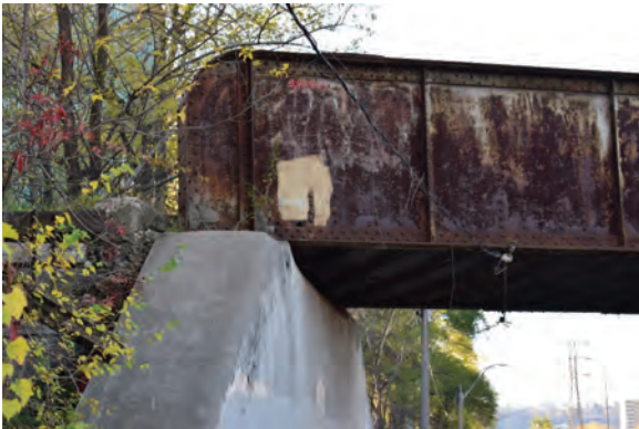
Plate 22: View of steel girders looking southwest
