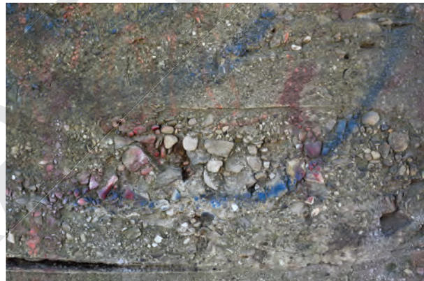
Plate 31: Close-up view of early concrete on west abutment
