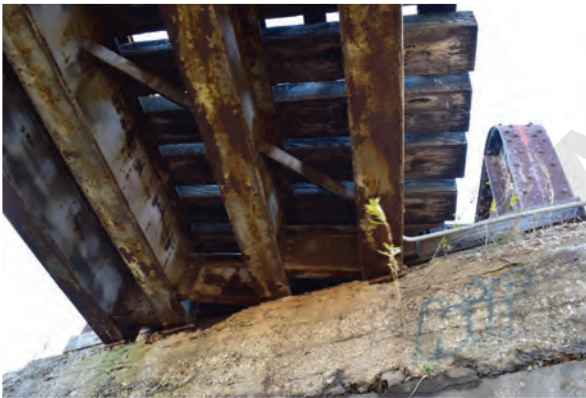
Plate 30: View of underside of railway line at west abutment looking southeast
