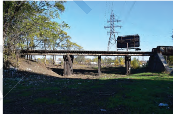
Plate 13: View of timber trestles looking northeast
