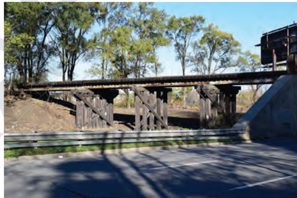
Plate 21: View of adjacent timber trestles looking northeast
