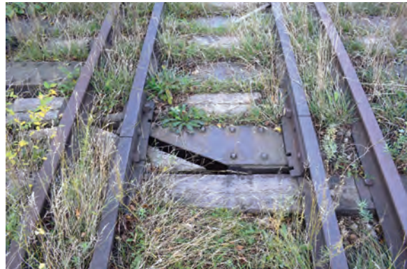
Plate 17: Close-up view of railway tracks over Birch Avenue Bridge
