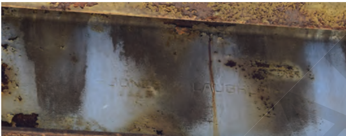
Plate 6: Jones & Laughlin inscription on middle steel beam of timber trestle
