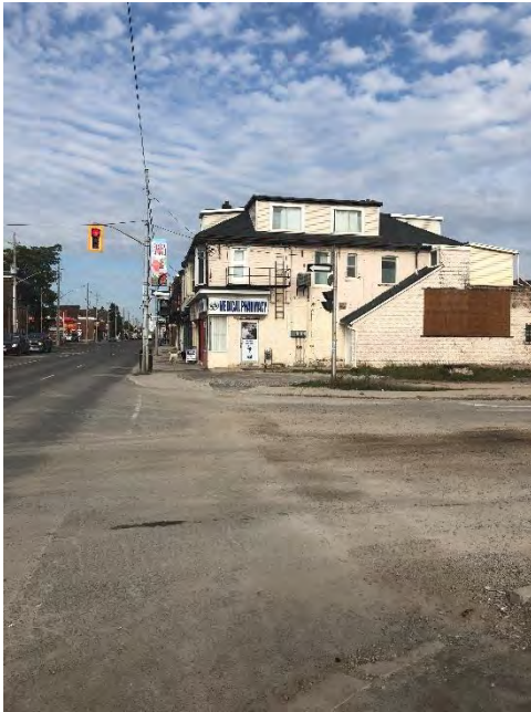
Plate 1: Intersection of Birch Avenue and Barton Street East, looking west towards 595 Barton Street East.
