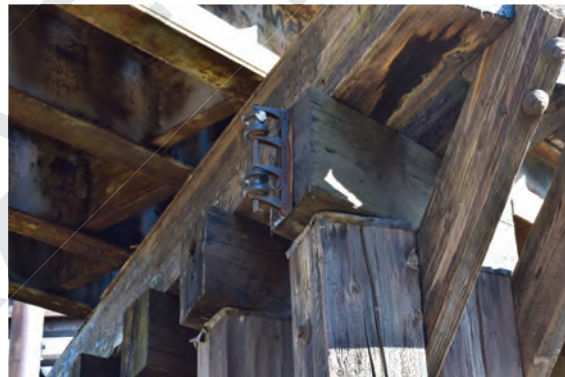
Plate 37: View of secondary rack on timber trestle
