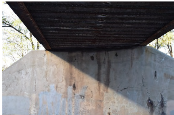
Plate 27: View of top of northwest abutment and steel girder
