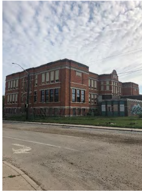
Plate 2: View of the former Gibson School, looking northeast.
