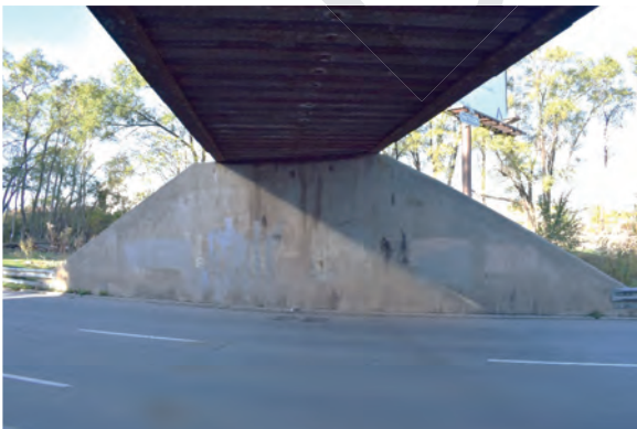
Plate 26: View of west abutment looking northwest
