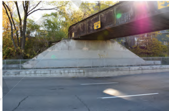
Plate 25: View of east abutment looking south
