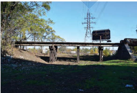
Plate 32: View of timber trestles looking northeast
