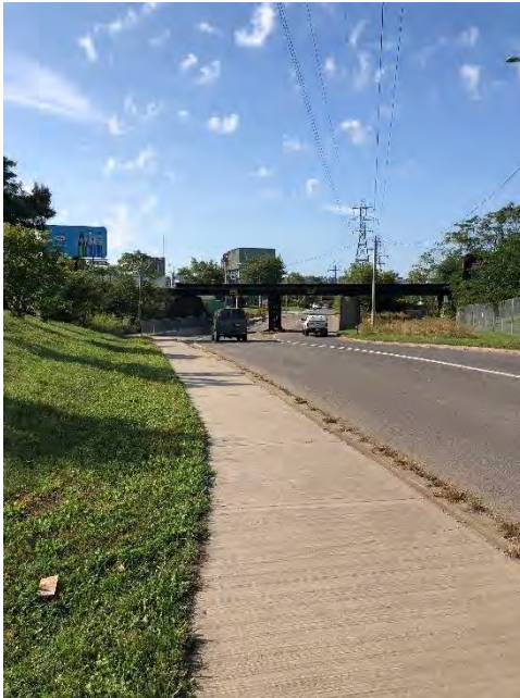
Plate 21: Bridge 330, looking south at Birch Avenue from Burlington Street East.
