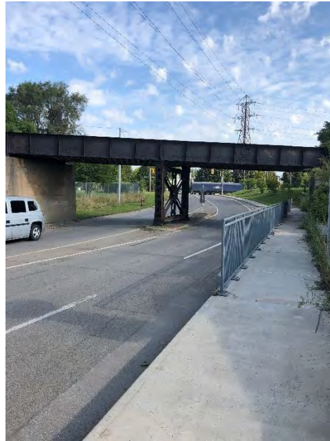
Plate 18: Northern railway crossing in the study area (Bridge 330), looking north.
