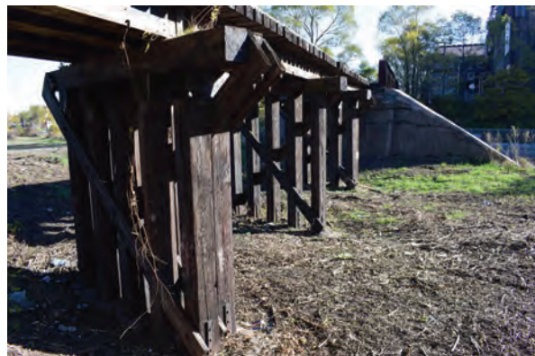
Plate 33: View of timber trestles looking southeast
