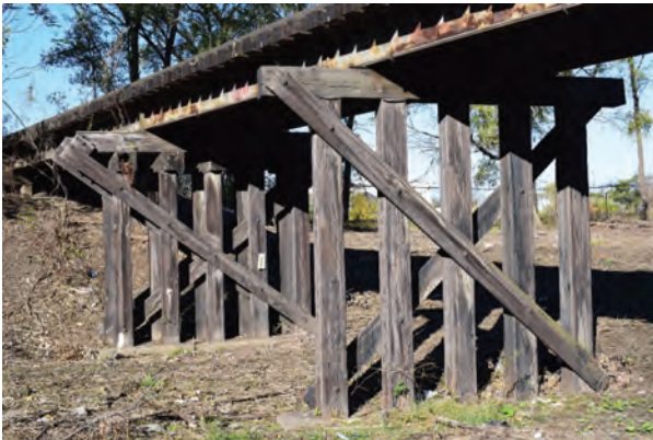
Plate 34: View of timber trestles looking northwest
