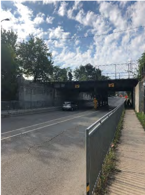
Plate 9: G.W.R. Main Line (Bridge 332), looking south.
