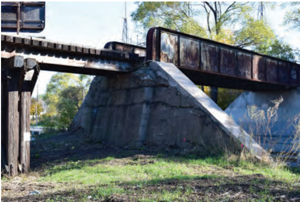
Plate 28: View of west abutment looking southeast
