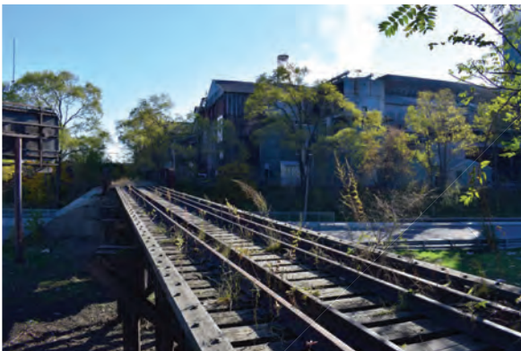
Plate 18: View of railway track across trestle support looking south
