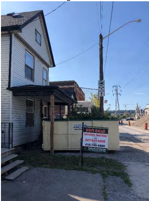
Plate 23: 156 Birch Avenue and in the distance the former school, looking south.
