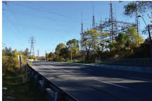
Plate 11: View of bridge approach looking northeast along Birch Avenue
