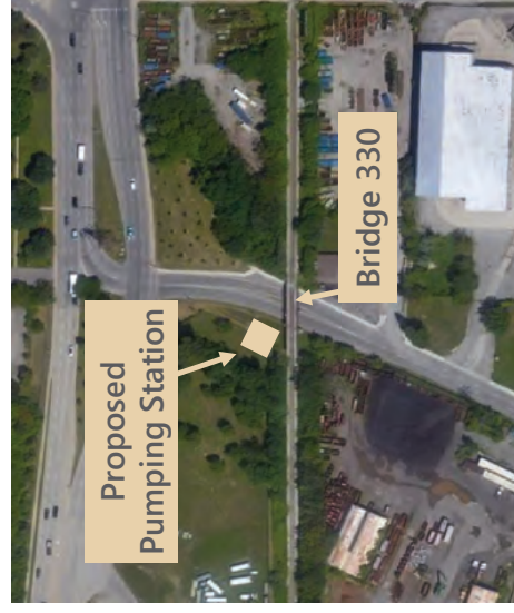
Proposed location of the Bridge 330 pump station.
