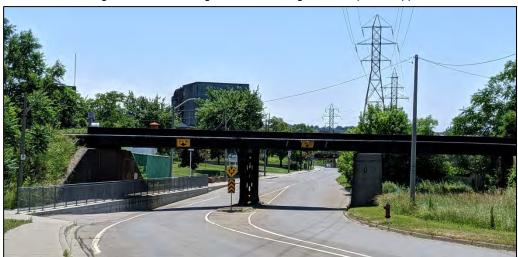
The structure is generally in poor to fair condition with moderate-severe corrosion and rust jacking of various members of the steel pier; severe rusting at the north girder's west end with perforation hole, local repair works on the girders and steel bent indicate the previous impact damages on these elements; as well as localized delamination/spall on the concrete pier and abutments.
