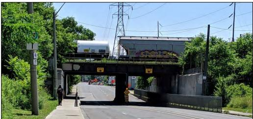
The structure is generally in fair condition with minor impact damage to the girders and gusset plates, severe corrosion on the bottom flange of the floor beam near the west abutment, structural steel coating failure, and, localized delamination/spall on the concrete abutments.
