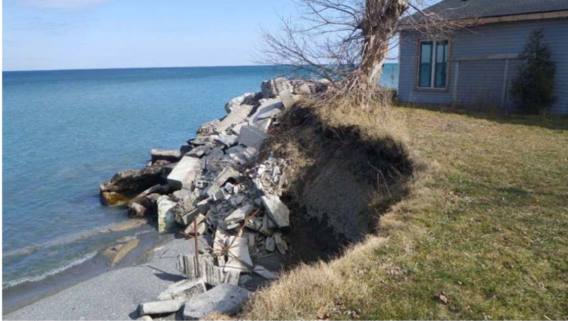
Figure 2.2: View of Headland at East End of Study Area
