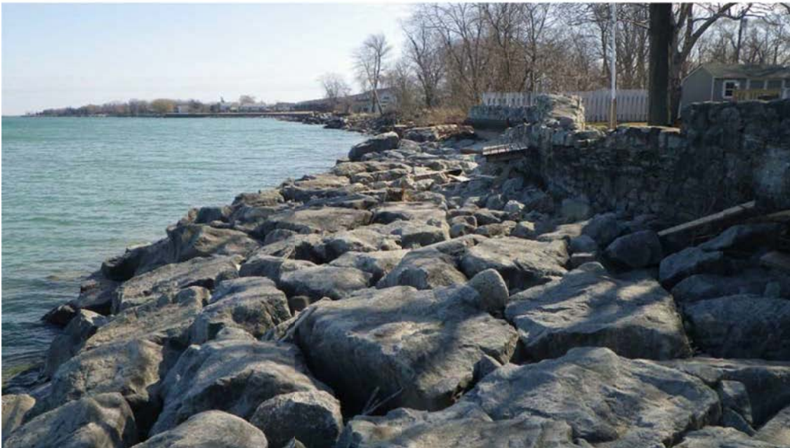
Figure 2.5: View from Adjacent Property to the West, Looking East
