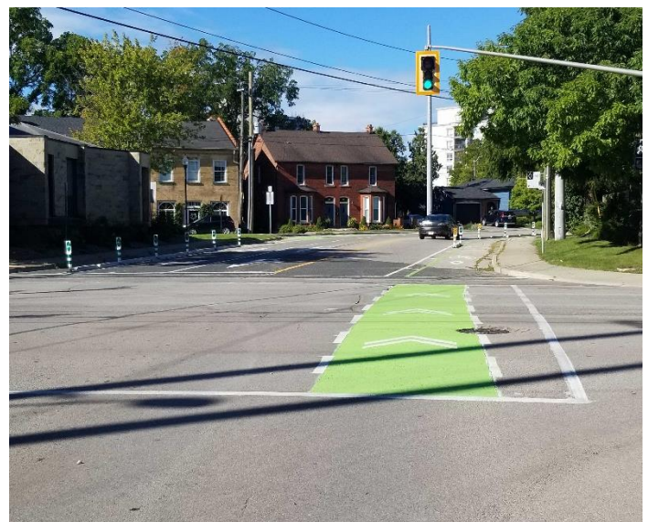
Hatt St @ Main St, Dundas Pavement markings
