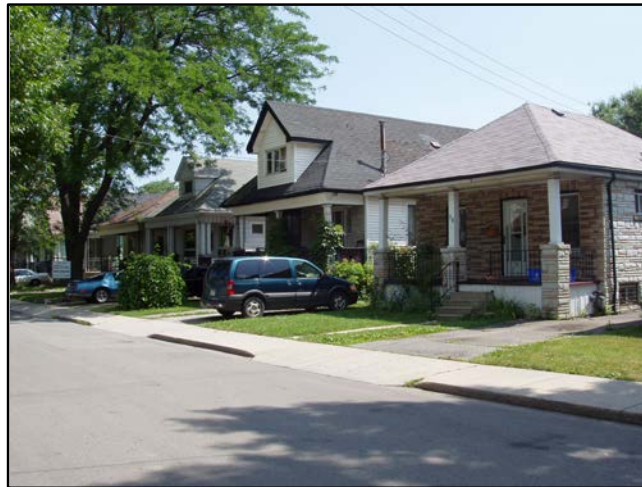
East Hamilton homes affected by storm damage. Huxley Avenue, south of Main Street. July, 2006. Photo Credit: City of Hamilton.
