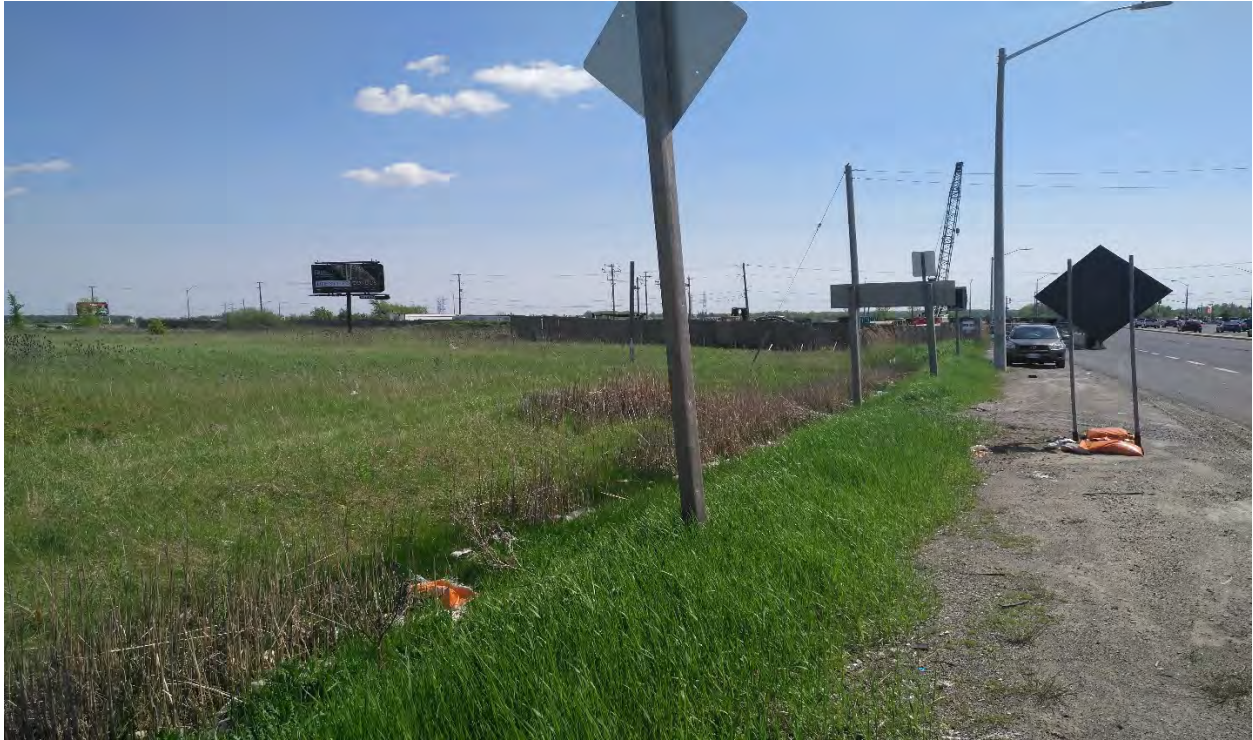
PS Site 1: Looking from Upper centennial Pky to south to Rymal Rd East, a view of the site vicinity with an ongoing construction project right at the northeast corner of the intersection.
