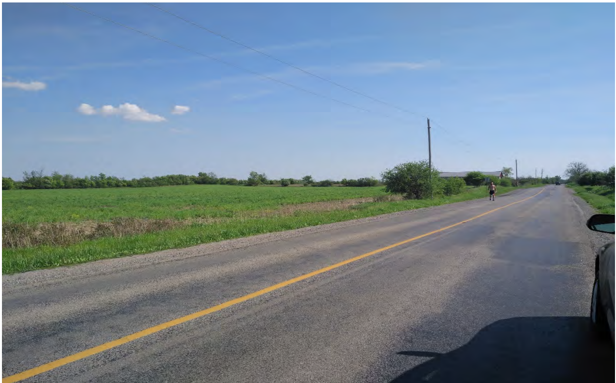
EWSF Site 2: A view from north to south on the east of Fletcher Rd, showing the site is a vacant farmland with vegetation growth and relatively flat grade
