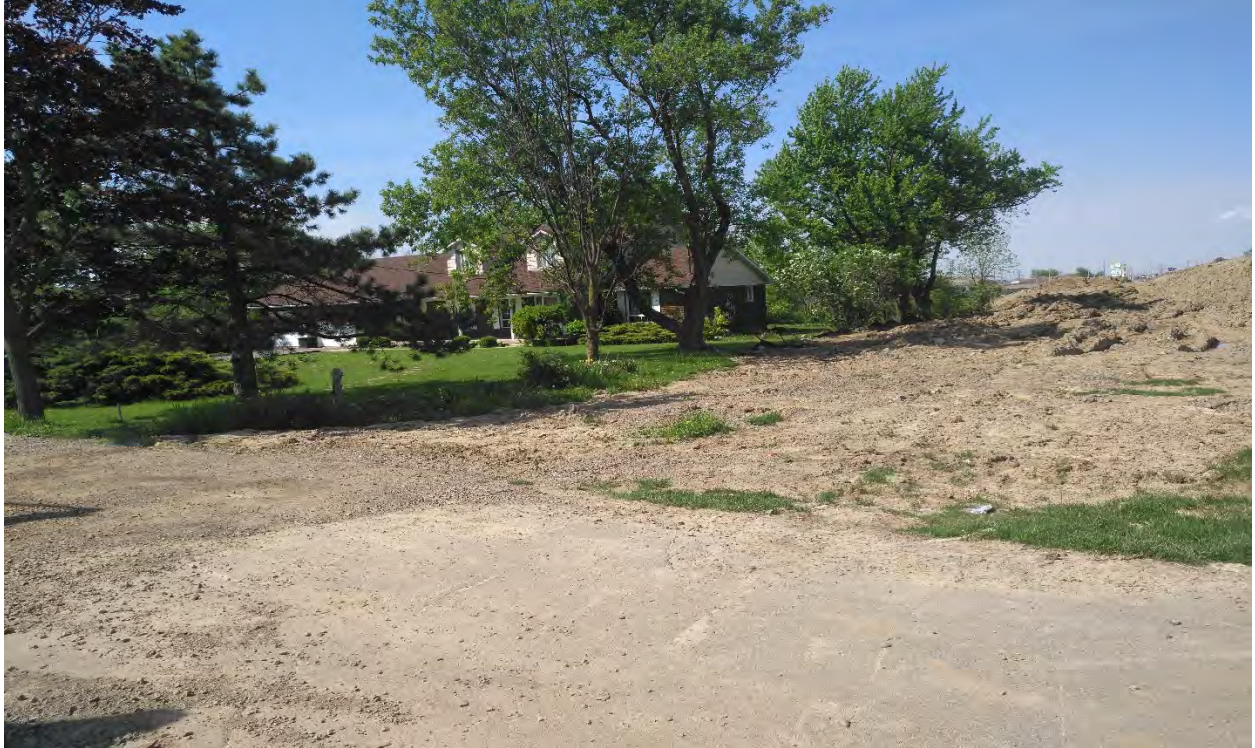
PS Site 3: A view from south to north, showing a residential property facing Rymal Rd East and soil stockpile generated from the construction site on its east and north sides.
