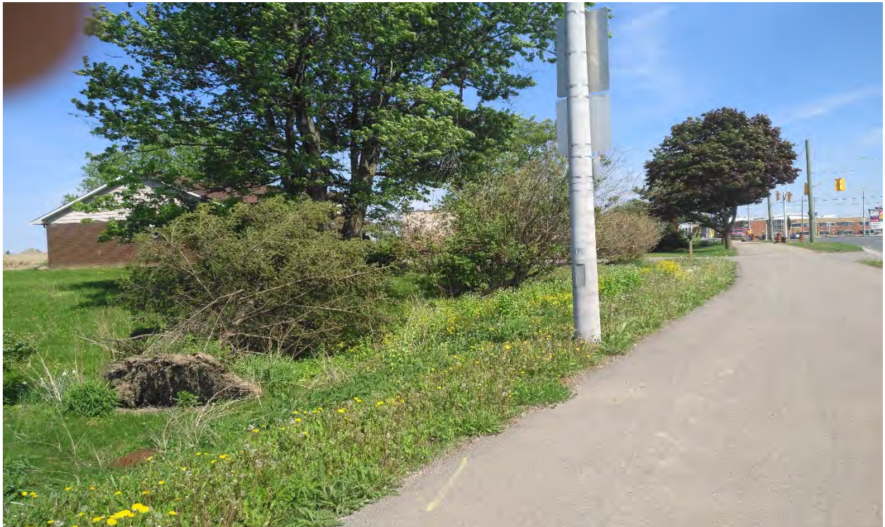
PS Site 3: Another view of the site from mid-west to east, showing the house and varied grade with the construction site on east of it.
