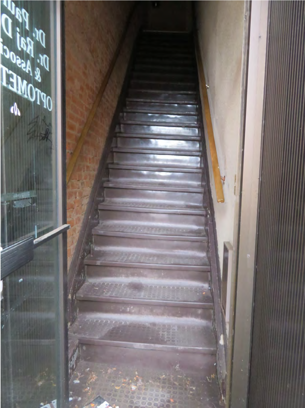
KING STREET ENTRANCE 2 – separate entrance for 2 nd floor tenant – 19 th century wood trim indicates an original staircase – the treads and risers have been clad in vinyl
