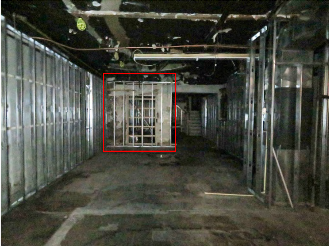
1 st FLOOR – rear section – this area has been gutted – note the exterior wall of a 19 th -century brick outbuilding that was integrated into the rear addition when it was enlarged sometime before 1911
