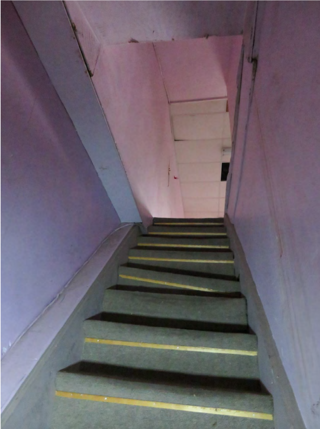
ATTIC STAIRS – steep staircase to the attic with no handrails – evidence of rot in the stair treads & stringer
