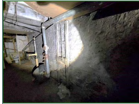
Photo 10 - Unit 164 - Basement wall collapse
