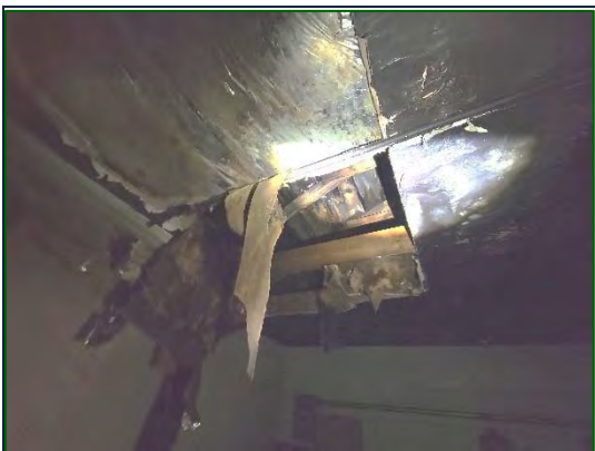
Photo 9 - Unit 164 - Ground floor ceiling collapse
