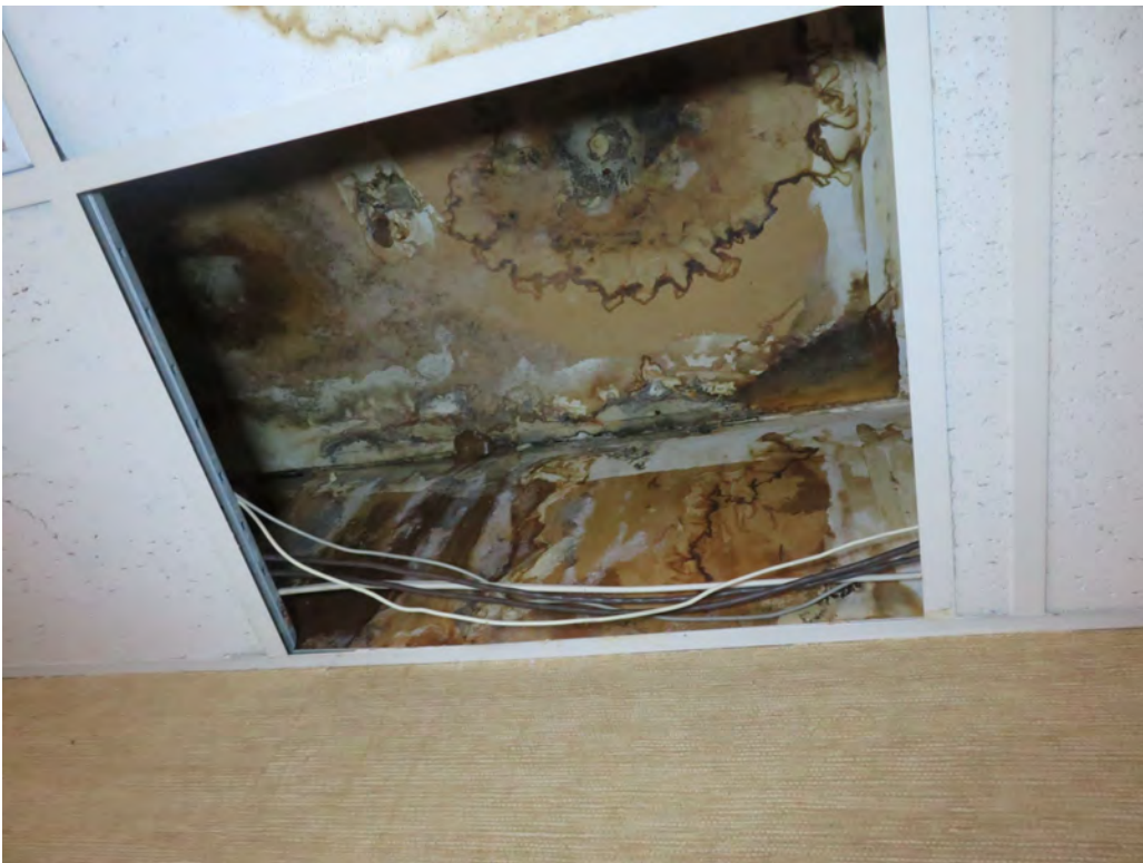
2 nd FLOOR DENTAL OFFICE – evidence of water damage and mould above the acoustic tile ceiling
