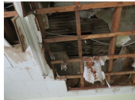
SATURATED INSULATION & COLLAPSED CEILING TILES
