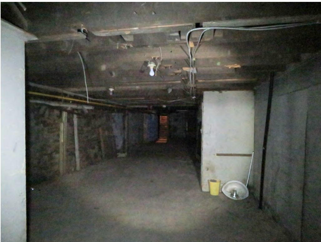
BASEMENT – unfinished basement – rubblestone foundation and floor framing date from the 19 th century
