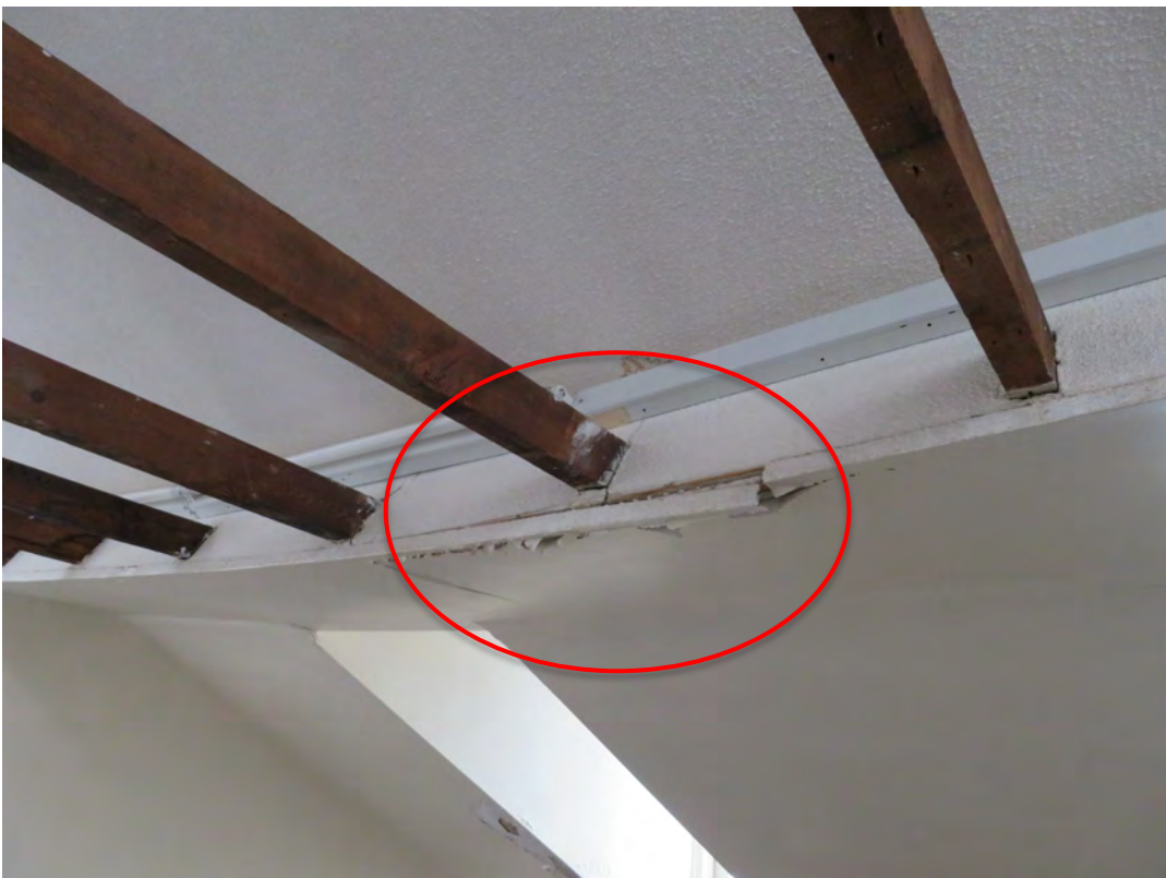
ATTIC – evidence of structural issues that has cause deflection of structural beams
