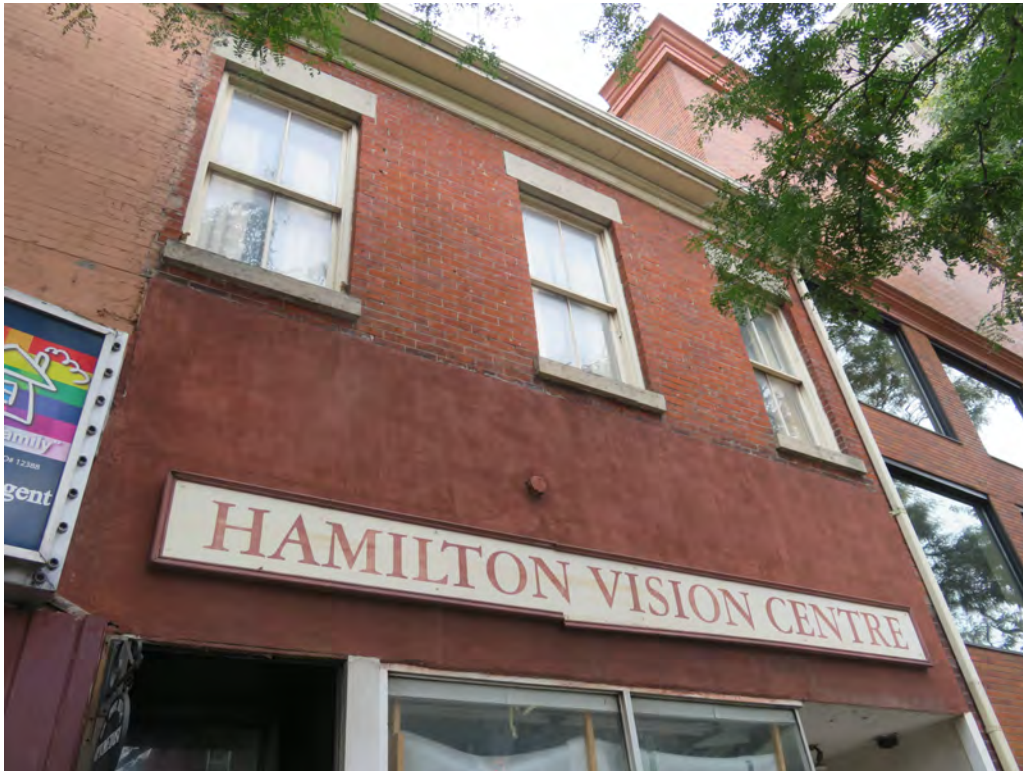
MAIN FAÇADE – original exterior wall with three window openings is partially intact on the 2 nd floor – the masonry below the 2 nd floor windows has been parged over – the original 2 over 2 wood sash windows remain
