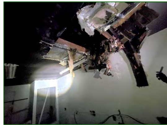
Photo 8 - Unit 164 - Ground floor ceiling collapse
