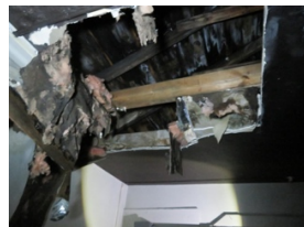
SATURATED INSULATION & COLLAPSED CEILING TILES
