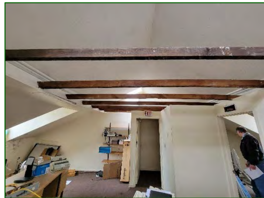
Photo 14 - Unit 164 - Third floor - rotated roof beam
