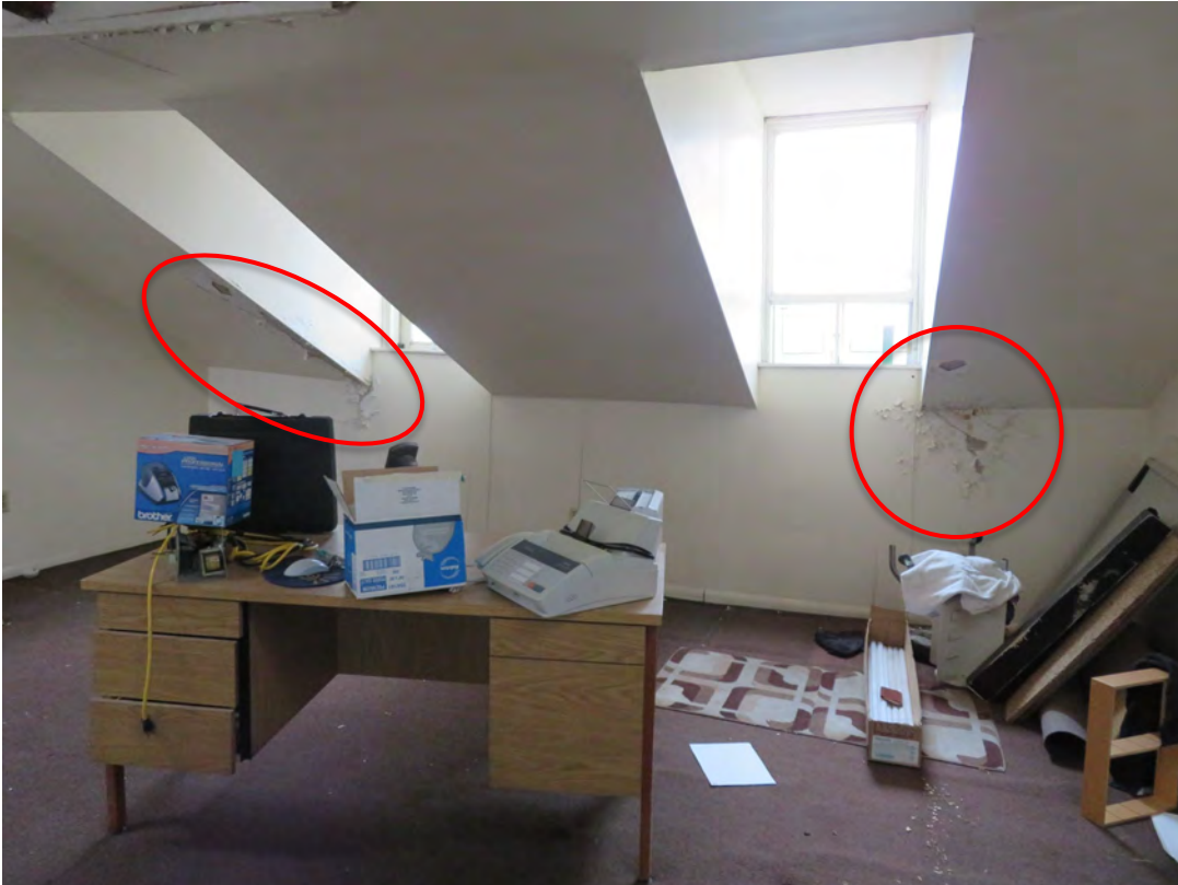
ATTIC – evidence of water damage around the roof dormers – no historic fabric
