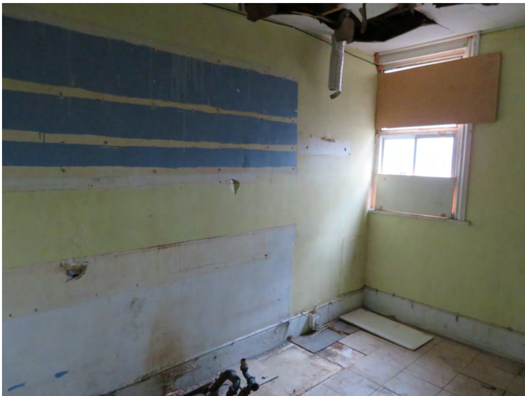
2 nd FLOOR KITCHEN – window trim is late 19 th century – evidence of extensive water damage to ceiling and floors
