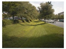
configured as a linear channel. The dry swale is a soil filter system that temporarily stores and then filters the desired water quality volume. Dry swales are similar to bioretention areas in that they rely on the same engineered media bed placed below the channel invert.
