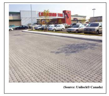
stormwater flows compared to traditional impervious paving surfaces like concrete and asphalt. Assuming the permeable designed paver is with adequate pretreatment and soil infiltration testing, a conservative runoff reduction rate of 90% is assigned to designs that rely upon full infiltration. Other benefits include reduce snow removal costs due to rapid ice melting and drainage, reductions in urban heat island effect (pavers have less thermal conductivity and thermal capacity
