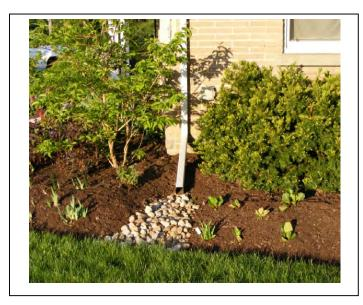
Rooftop disconnection with treatment is possible on lots with any size and configuration; however functional downspout disconnection requires a minimum length of pervious flow path and appropriate soil conditions.
