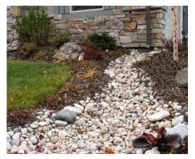
The amount of the water balance requirement met will depend on the amount of runoff stored and percolated into the native soils. Runoff reduction capability of soakaway pits, is presumed to be high, given that infiltration is the designed intent of the practice, however some surface overflows do occur when the infiltration storage capacity is exceeded. Assuming the practice is designed with adequate pretreatment and soil infiltration testing, a conservative runoff reduction
