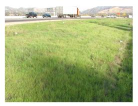
peak discharge by maintaining runoff in sheet flow, thereby resulting in a longer time of concentration.
