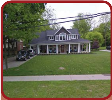
Characteristic Gateway Residential Building
