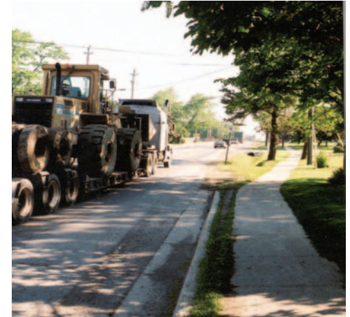
There is little separation between the traffic and the sidewalk creating an uncomfortable and dangerous atmosphere for pedestrians. The 1.2m wide sidewalks in the core are generally undersized and lack any pedestrian amenities.
