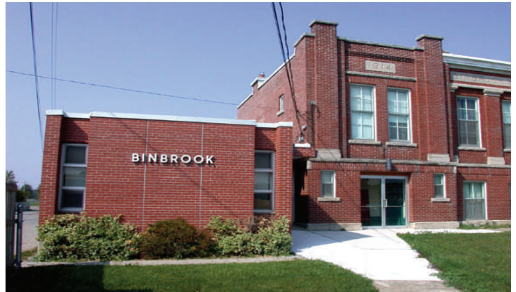
The addition to the Binbrook Memorial Hall is an uncomfortable fit both in its location and height. While an effort was made to match the existing brick type and colour, the forward placement of this addition detracts from the grandness of the existing building. Following the advice in these guidelines may assist in selecting better locations and building forms.
