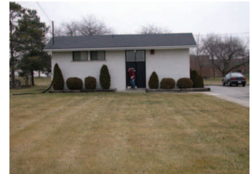
Existing medical office with front lawn and side yard parking .
