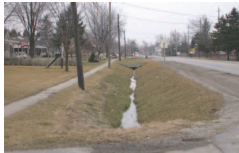
Highway 56 south of the main intersection. Note the gravel shoulder and open ditch.
