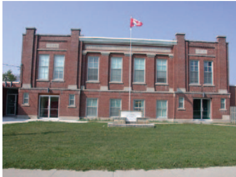
The Binbrook Memorial Hall constructed in 1920 is one of a few historic buildings of great prominence within the community core. Opportunities to incorporate this building into the Binbrook streetscape are numerous.
