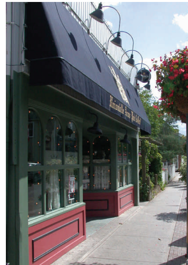
The renovated storefront on this building incorporates the principles of good storefront design; ample window area to provide good retail exposure, a recessed doorway, and front lit signage on the awning.
