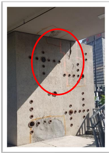
Figure 1: Partly Damaged Column and Slab
