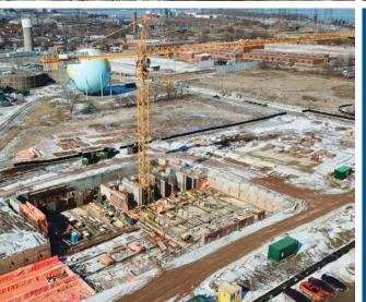
Demolition of the Aeration and Clarifier tanks for phase 1 construction is complete and modifications to these structures commenced, beginning with piles and lagging being installed. Concrete work continued for the Tertiary Facility and removal/installation of underground utilities is ongoing. In addition, a tower crane was erected to aid in commencing the construction of the Tertiary Facility. Excavation started on the Chlorine Contact Tank.
