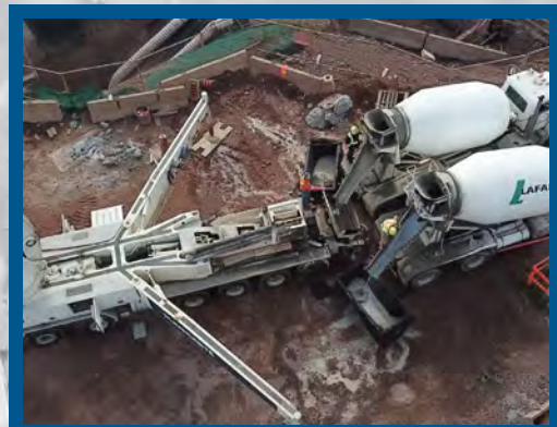
240 truckloads of concrete
