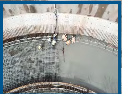
2092m 3 of concrete 1.3-1.4 metres thick
