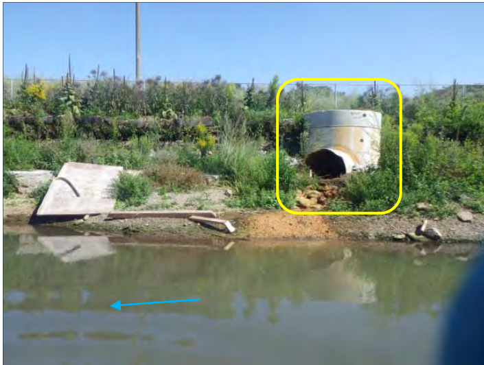
Facing culvert located upstream of sample transect on east bank.
