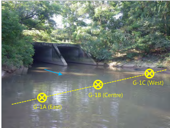
Replicate grab locations at transect G-1 downstream of culvert.
