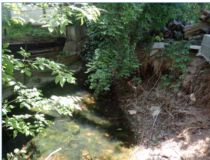
Figure 5-1: Watercourse 6.0, downstream end (June 9 2016)
