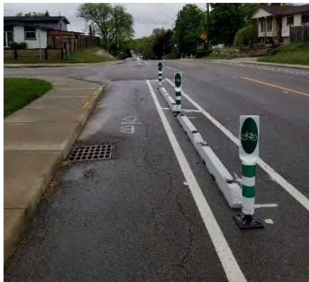
Upper Paradise Rd, Hamilton Buffered bicycle lanes with barriers
