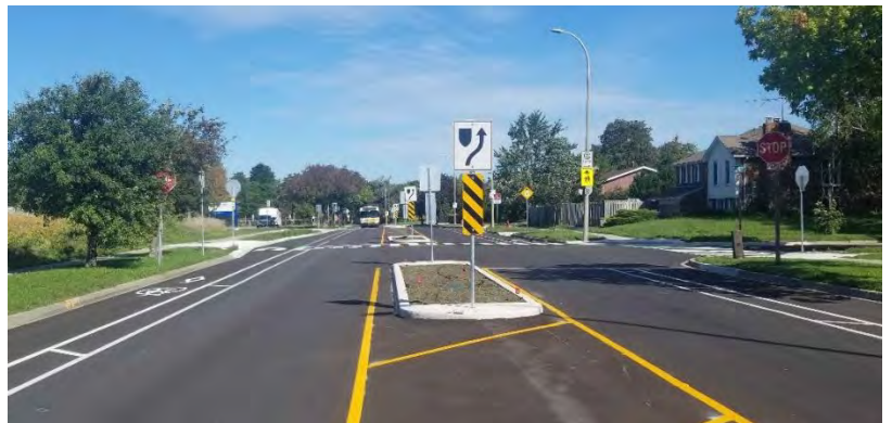
Paramount Rd, Hamilton Buffered bicycle lanes
