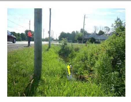
The Barton Street crossing appeared to be causing a slight backwater, as evidenced by the standing water upstream of the structure.
