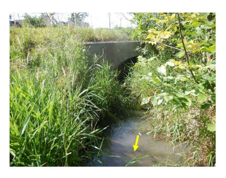
The crossing at Barton Street was a circular concrete culvert which had been partially blocked by riparian vegetation which had colonized the channel.
