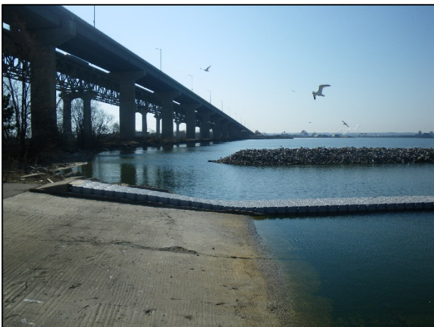
East shoreline of Hamilton Harbour facing south. Note boat launch in foreground and Burlington Skyway to left
