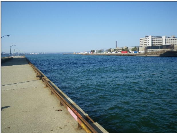
West portion of the Burlington Canal facing west into Hamilton Harbour
