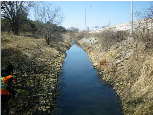
Eastport Ditch 1 facing upstream (NW) from outlet culvert
