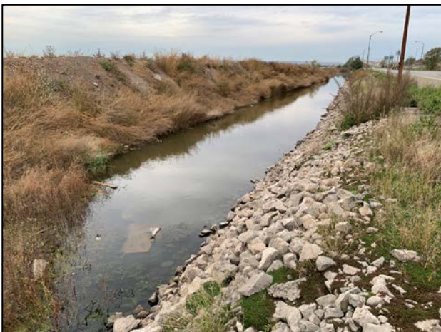
North portion of Eastport Ditch 3, facing northwest (November 2021)
