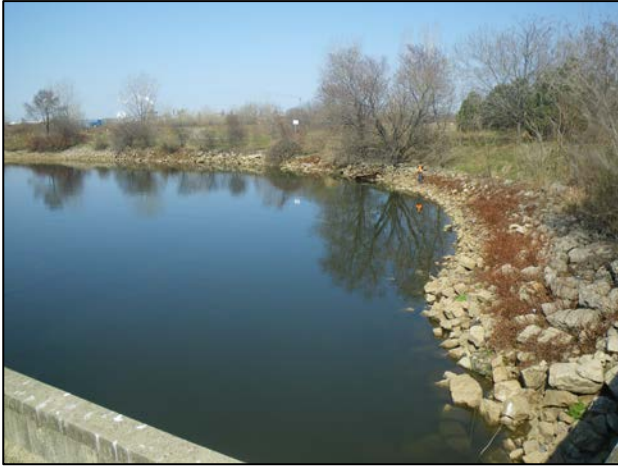
Upstream end of Red Hill Creek facing downstream (NW) from Eastport Drive crossing. Note CSP outlet from Eastport Ditch 1 along shoreline
