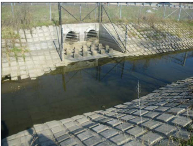
Outlet from storm water system of Beach Boulevard community, facing east
