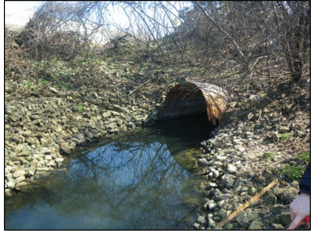
Upstream end of outlet to Red Hill Creek, facing SE
