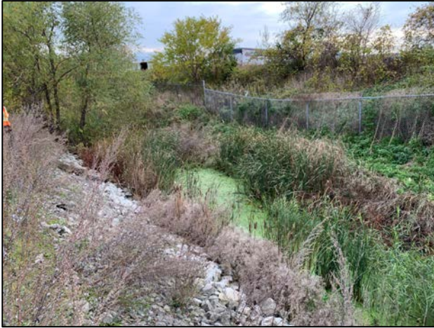
South end of Eastport Ditch 3 at end of growing season. Facing south
