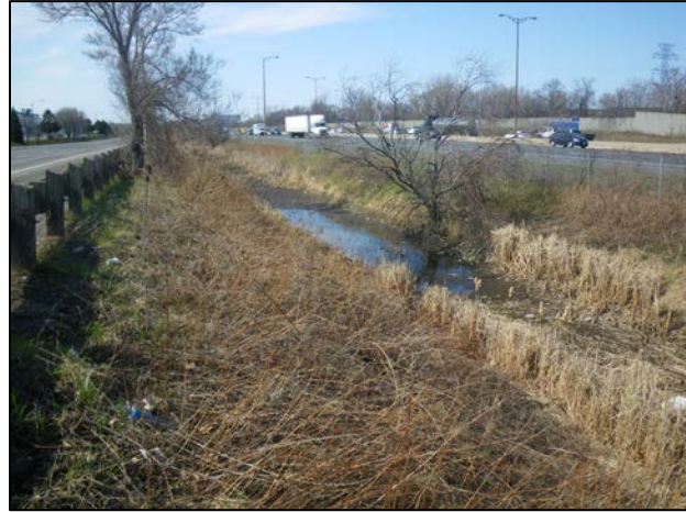
Downstream portion of Eastport Ditch 2, facing upstream (NW)
