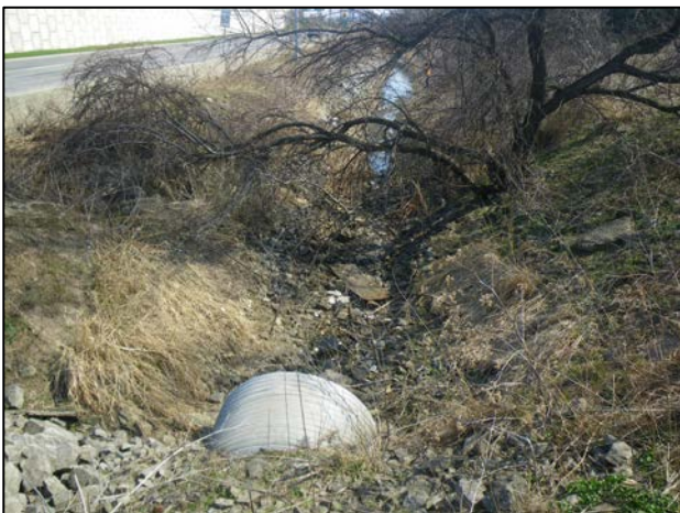
Downstream end of outlet pipe from Eastport Ditch 2, facing downstream (SE)
