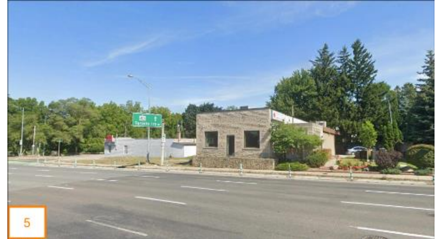
Figure 6: Existing buildings within the development area.
