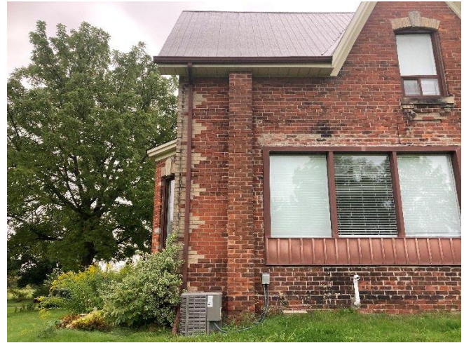
Plate 41: Remnants of a second brick chimney on the west elevation. Large breach on west elevation to accommodate new window.
