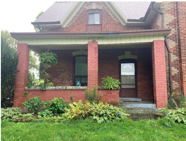
Plate 42: Veranda with brick piers and half walls with stone coping on front facade
