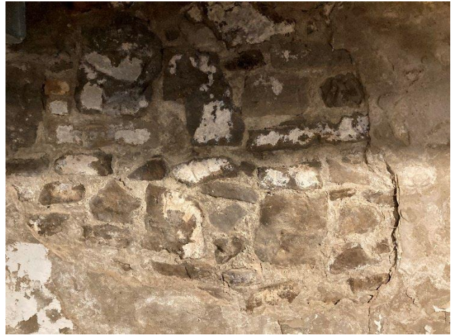
Plate 67: Course rubble foundation covered in plaster
