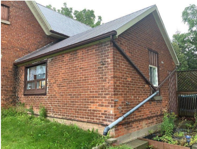
Plate 44: Rear addition set on poured concrete and clad in red brick in stretcher bond
