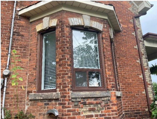
Plate 38: East bay window with segmental arch head and keystone and stone sill with recessed buff brick detailing
