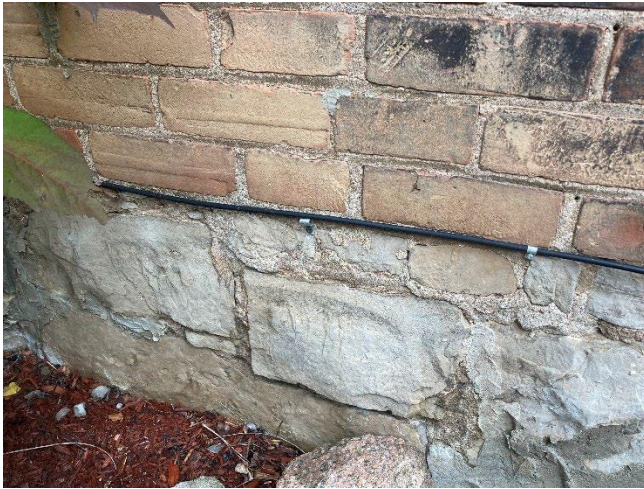
Plate 36: Coursed rubble foundation on east elevation
