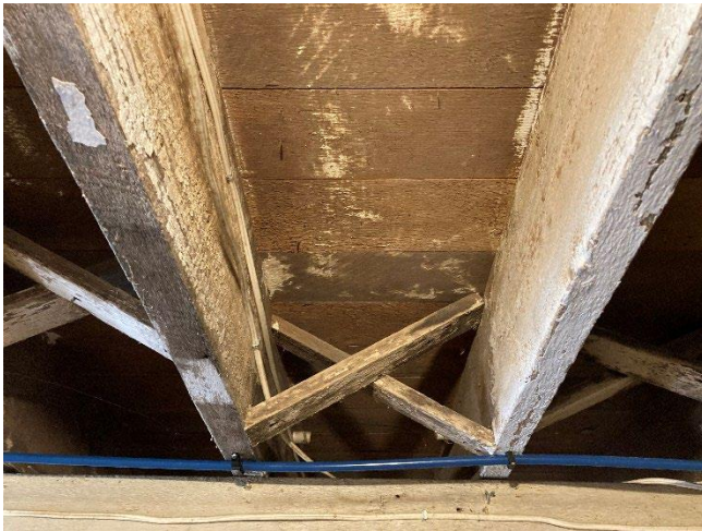
Plate 72: Circular sawn floor joists for the ground floor
