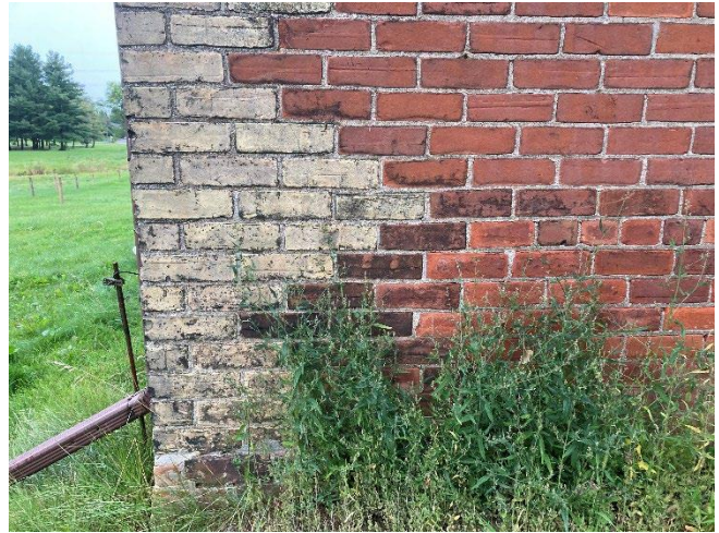
Plate 37: Buff brick diamond quoin and water table on south elevation
