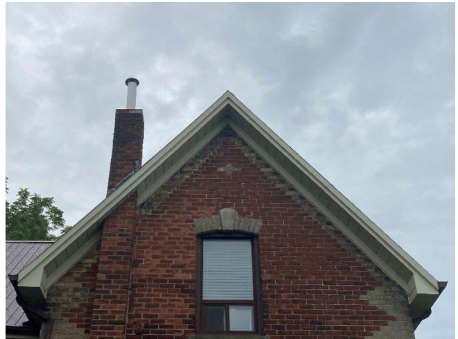
Plate 39: Buff brick staggered Flemish bond border and detailing in the north elevation gable
