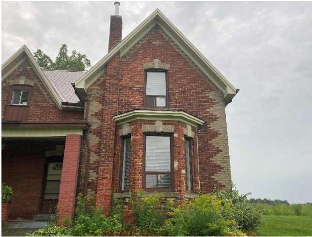
Plate 40: Exterior single-stack brick chimney on the front or north façade
