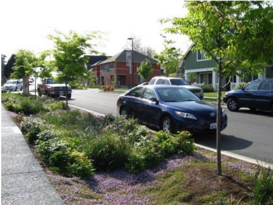
Figure 8: LID BMP Conveyance Swale
