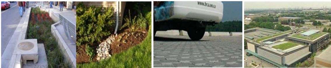
(From L to R: Special Bioretention, Downspout Disconnection, Permeable Pavement & Green Roofs)
