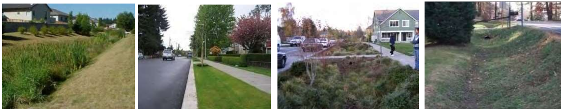
(From L to R: Vegetated Channel, Subsurface Perforated Pipe, Bio-swale & Grass Channel)
