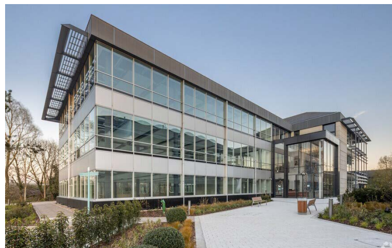
Fig. 3.8.6 - Image example of rooftop mechanical equipment screened from ground level view through integration with roof form.
