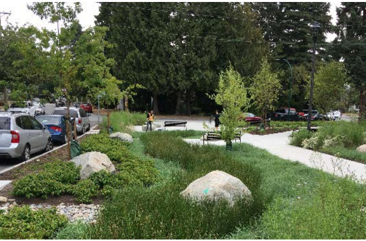
Fig. 3.10k - Image example of a bio-retention swale for managing storm water runoff.
