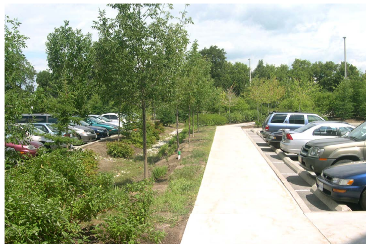
Fig. 3.10p - Image example of parking area with integrated LID (bio-retention swales).
