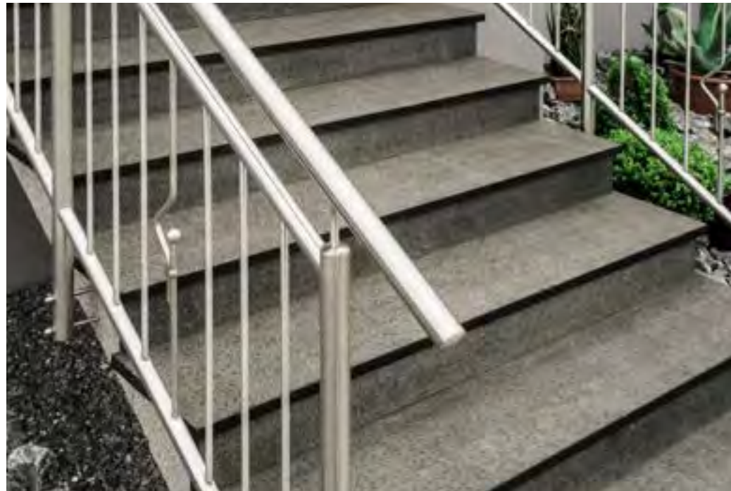
04 EXISTING STEEL STAIRCASE CLAD WITH NON-SLIP GRANITE ON BOTH TREAD AND RISER
