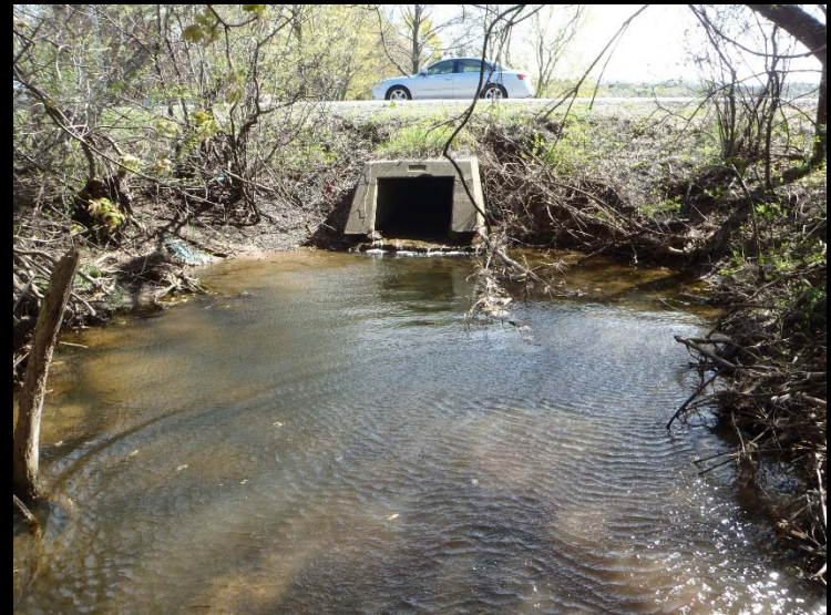
Photo 24: WC 7.1, downstream, end of crossing.
