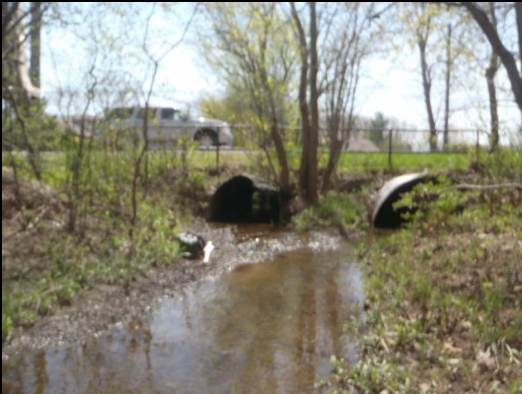
Photo 11: WC 6.0 standing at downstream end of culverts facing upstream.
