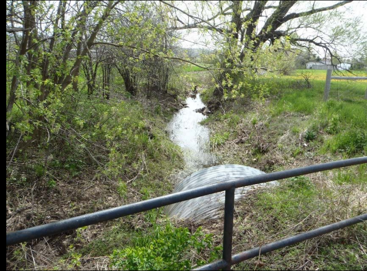
Photo 22: WC 7.0, at upstream end of crossing, facing upstream.
