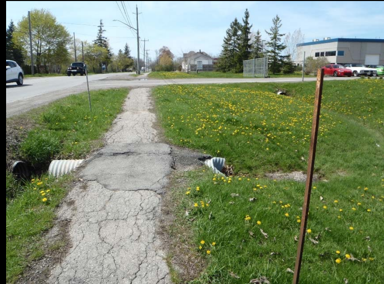
Photo 18: WC 6.1 downstream of crossing.
