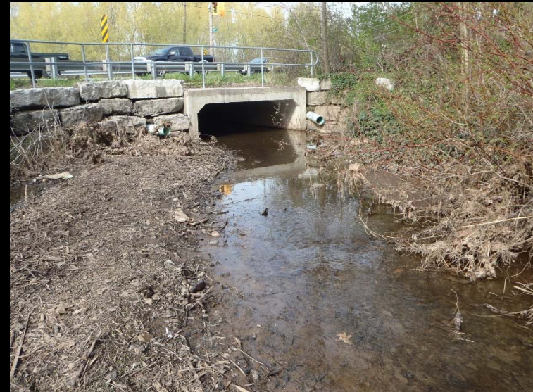
Photo 36: WC 12 upstream of crossing.
