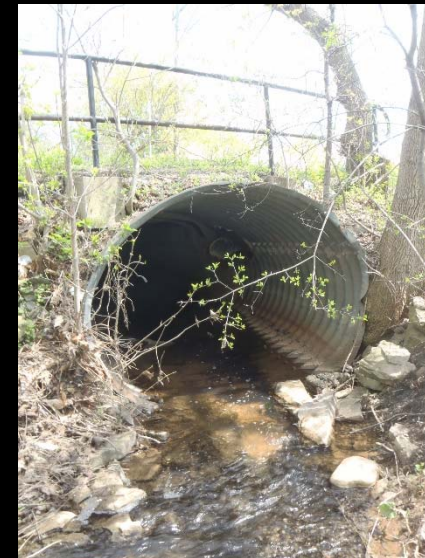
Photo 4: W 5.0 standing at upstream end of culvert facing downstream.
