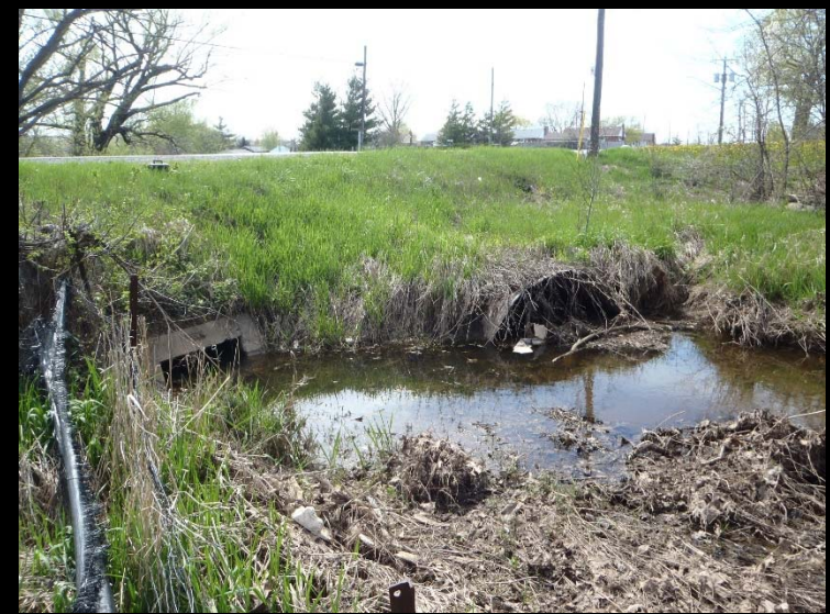
Photo 20: WC 7.0, downstream end of crossing.
