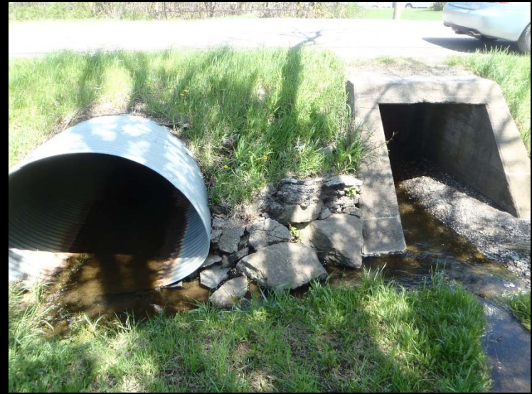
Photo 14: WC 6.0, upstream end of culverts.
