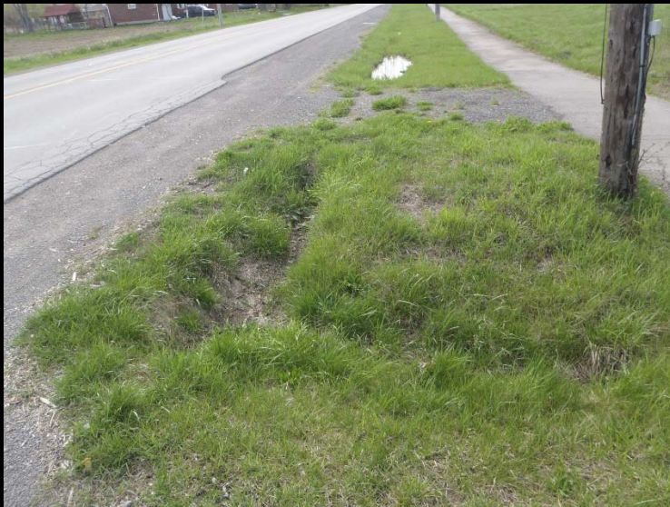
Photo 31: WC 7.2 at downstream end of culvert.
