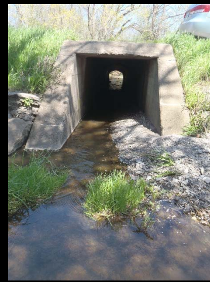
Photo 16: WC 6.0 within ROW.
