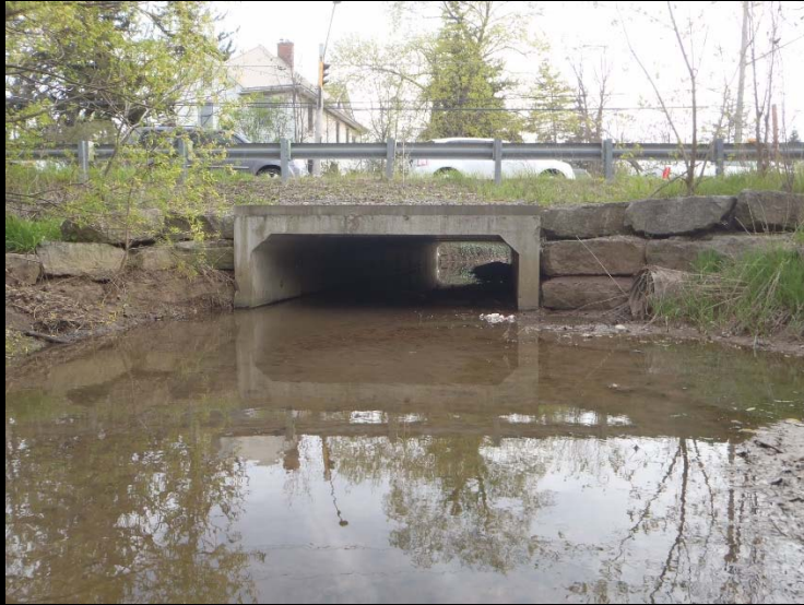
Photo 33: WC 12, downstream end of crossing facing upstream.
