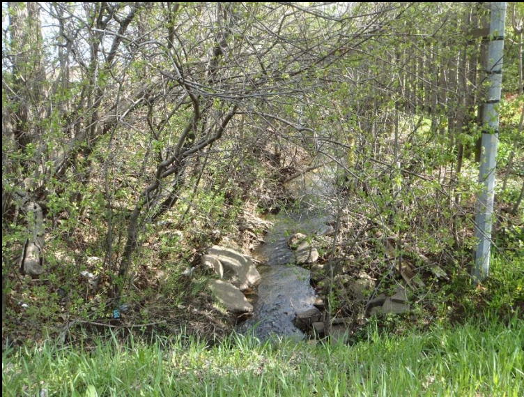
Photo 1: WC 5.0 facing downstream.
