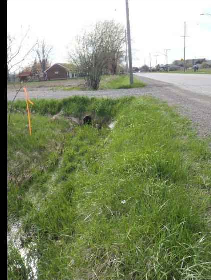
Photo 30: WC 7.2 at upstream end of culvert.
