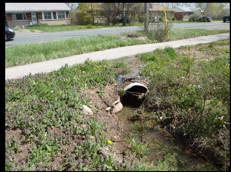
Photo 8: WC 5.2 standing at upstream end of culvert facing downstream.
