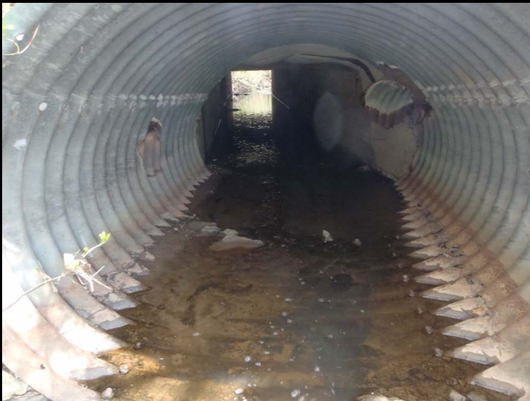
Photo 5: WC 5.0 within the ROW, facing downstream.
