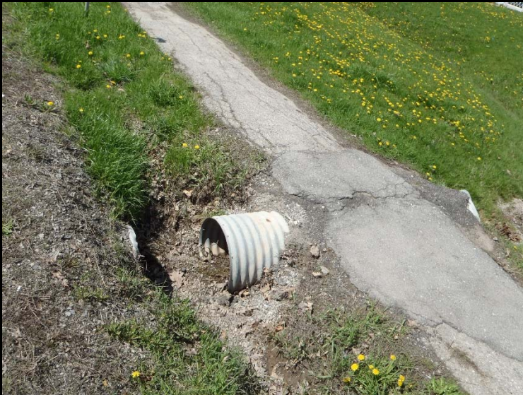
Photo 17: WC 6.1 upstream of crossing.
