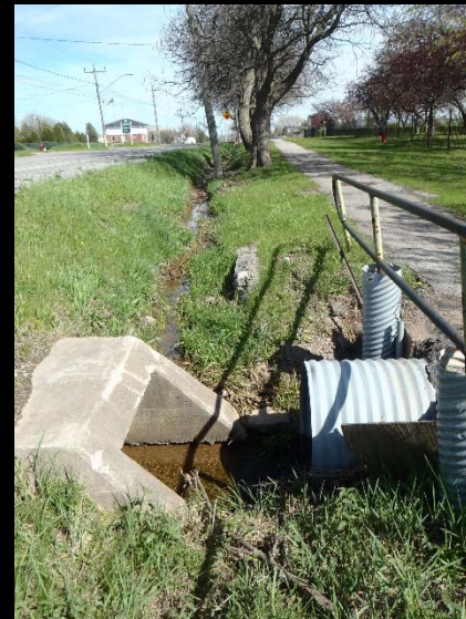
Photo 28: WC 7.1, merge point between two crossing structures.
