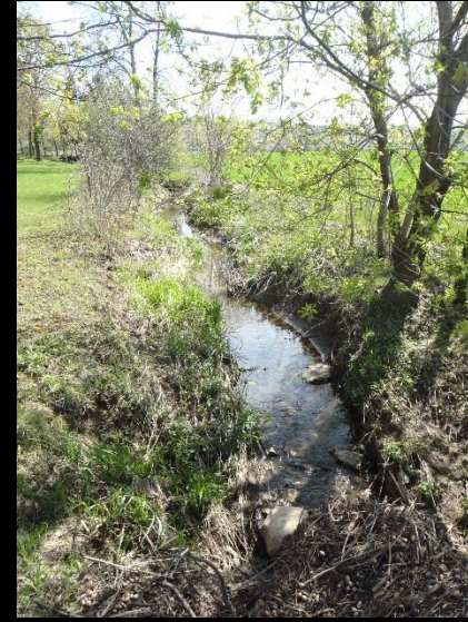
Photo 26: WC 7.1 at upstream end of crossing facing upstream.
