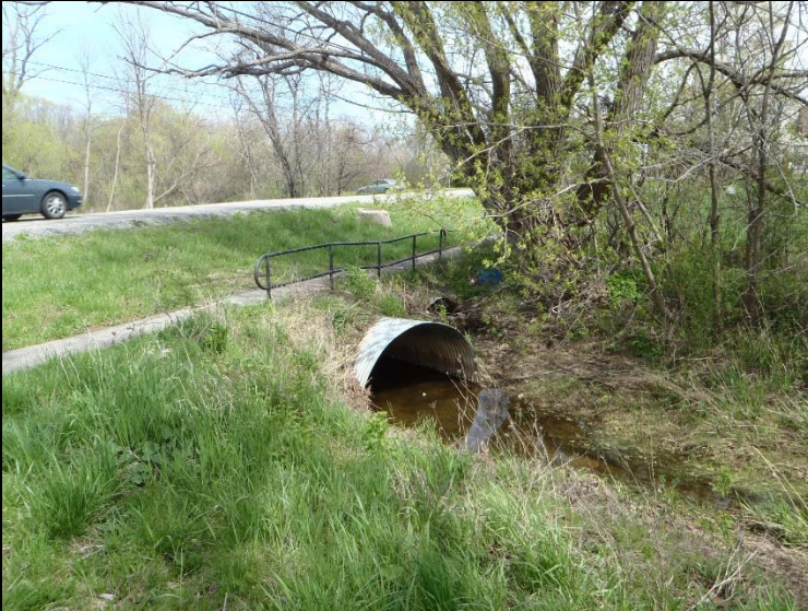
Photo 21: WC 7.0, upstream end of crossing.
