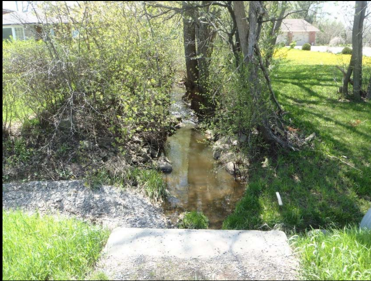
Photo 13: WC 6.0 standing at upstream end of culvert facing upstream.
