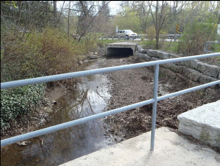
Photo 35: WC 12 upstream of crossing.
