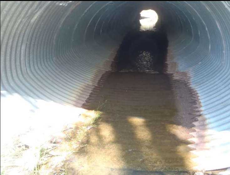
Photo 15: WC 6.0 within ROW.
