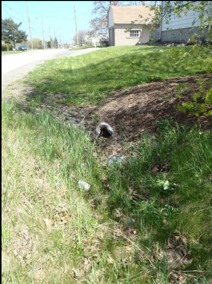
Photo 9: WC 5.2, downstream of crossing.
