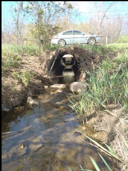
Photo 27: WC 7.1 at upstream end of crossing facing downstream.
