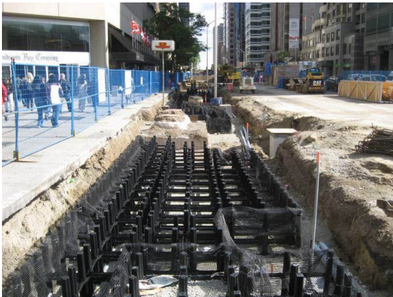
Figure 5.4 Silva Cell Construction ( www.smartcitiesdive.com , 2020)
