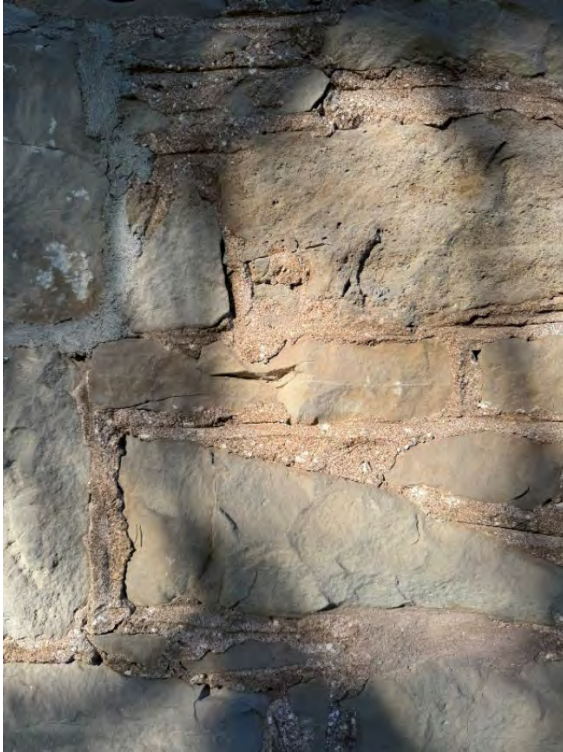
Incompatible Repointing of Limestone Façade
