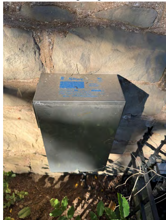
Low Voltage Transformer for Outdoor Lighting
